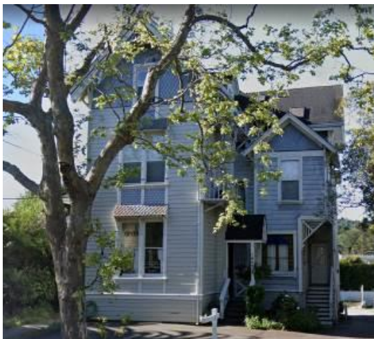
1607 5 th Avenue (011-196-02). Good example of stick-style residence. Included in 1978 survey. Rate as B.
