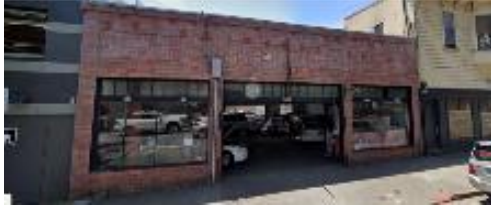
1117 3 rd Street (APN 011-262-25). Milani Garage. Located within eligible west district. Retain as “C” for future evaluation. No year of construction provided by Assessor..R
