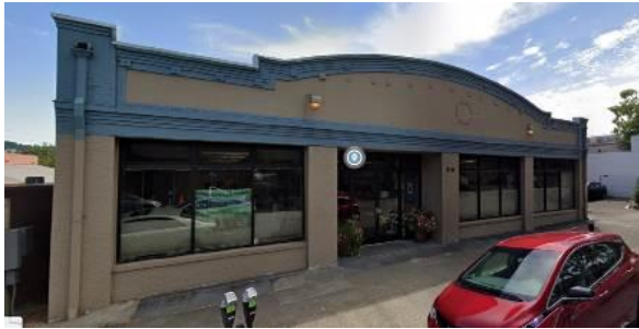
819 5 th Avenue (APN 011-224-13). Property already appears on a Fact Sheet as a Contributor (836 Fourth, Mikes Bikes--rated “B”) but this is the rear façade facing 5 th Avenue. This space has been repurposed and is now separate from the 4 th Street façade.
