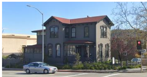
824 E Street (011-252-21). Residence converted to offices (Polaris/Greystone Financial Group). Future study recommended. No year of construction on record. Likely an "A" rated building.
