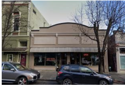
936 B Street (APN 011-261-01). This structure is on the same parcel as Mulberry House/ McDermott Building (938 B), which is a designated local landmark. The building at 936 was formerly a Quonset hut that was attached at the high side to the Mulberry House. It is rated "B" and is considered a contributing structure. Current use is Diamond Nails.
