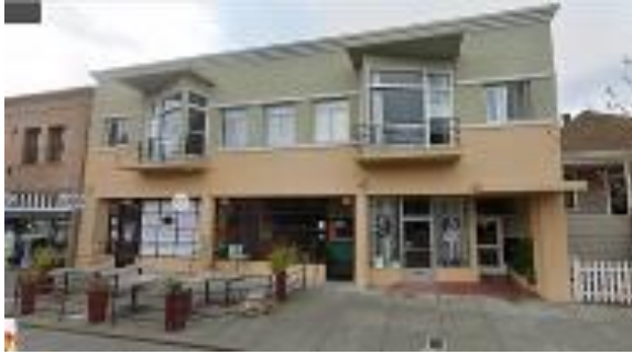
1559-1565 4 th Street (APN 011-242-03). Good example of an international style storefront. Retain as “C” for future evaluation.
