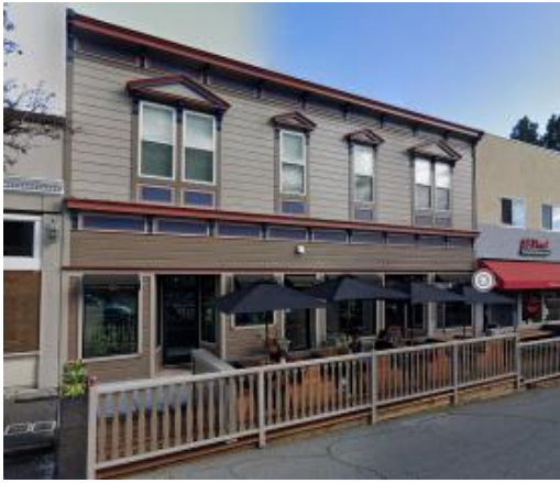
924 (920-926) B Street (APN: 011-261-12). Mash Building/ Butcher. M Herzog (now Libation Taproom). Contributing structure in the Eligible Downtown West historic district. Rated as B. Surveyors had questions about integrity of the recent remodel.
