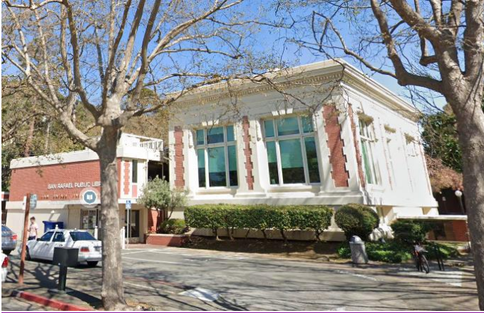
View of the original library structure and details and modern additions. (2019)
