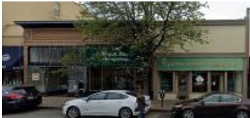
1318-1320 4 th Street (APN 011-205-10). Marelli Bros. Shoe Repair. Likely a contributor to the West Downtown Core eligible district. Intact 1880 storefront and transoms. Adjacent building on same parcel may have resulted in Fact Sheet not being prepared. Retain as “B.”
