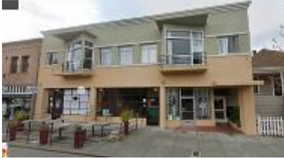
1559-1565 4 th Street (APN 011-242-03). Good example of an international style storefront. Retain as “C” for future evaluation.
