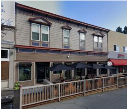
924 (920-926) B Street (APN: 011-261-12). Mash Building/ Butcher. M Herzog (now Libation Taproom). Contributing structure in the Eligible Downtown West historic district. Rated as B. Surveyors had questions about integrity of the recent remodel.
