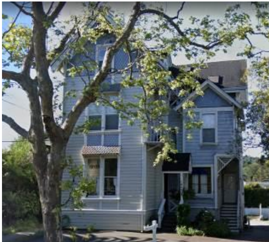
1607 5 th Avenue (011-196-02). Good example of stick-style residence. Included in 1978 survey. Rate as B.
