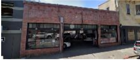
1117 3 rd Street (APN 011-262-25). Milani Garage. Located within eligible west district. Retain as “C” for future evaluation. No year of construction provided by Assessor..
