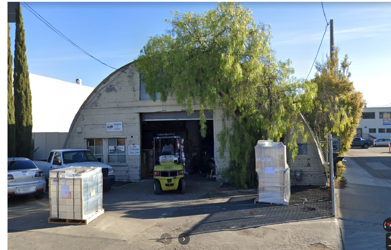
16 DeLUCA PLACE EXISTING BUILDING (TO BE REMOVED)
