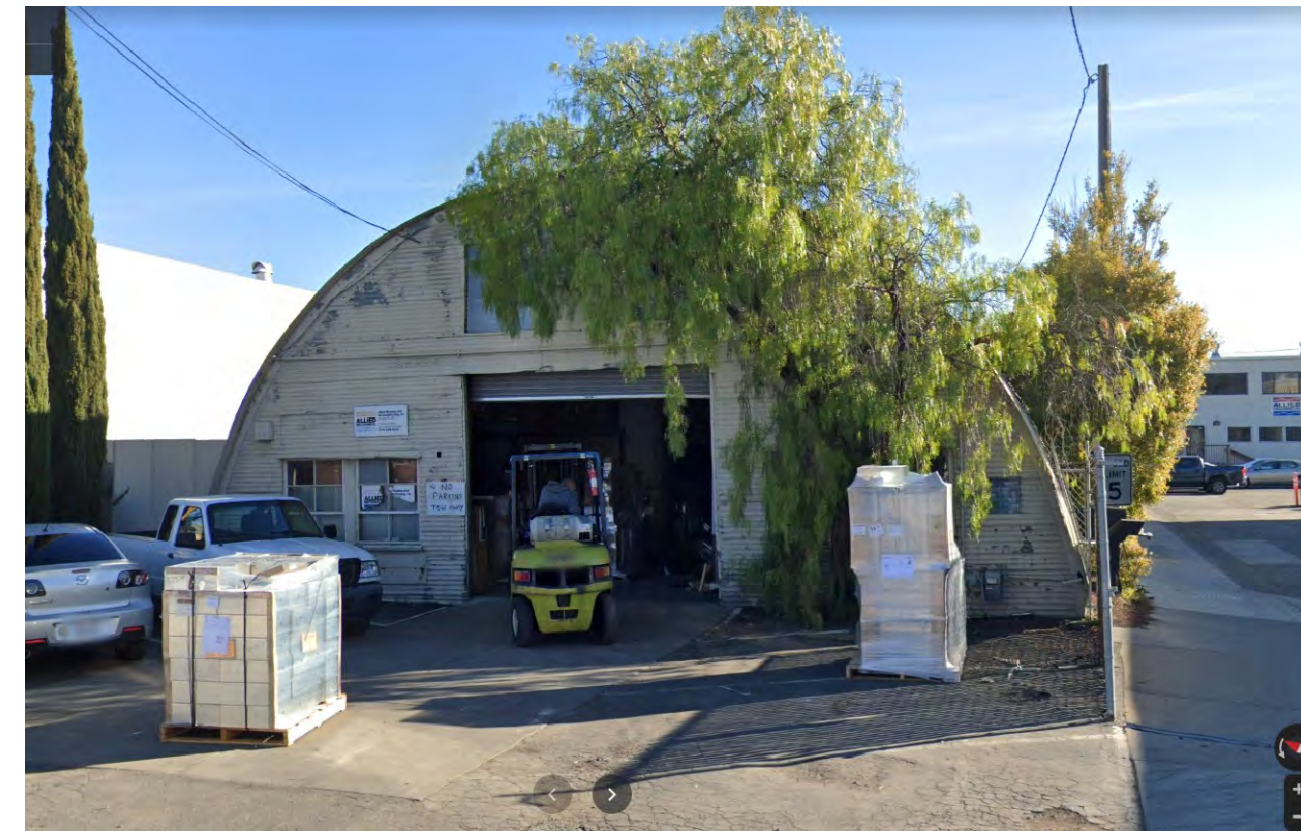
16 DeLUCA PLACE EXISTING BUILDING (TO BE REMOVED)
