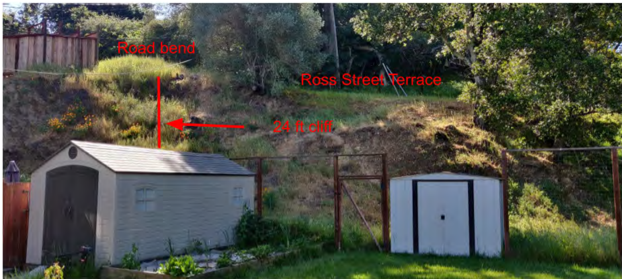
Figure 1. View of the Ross Street Terrace from my house at 211 Marin St. Road bend and a 24 ft cliff are shown.
