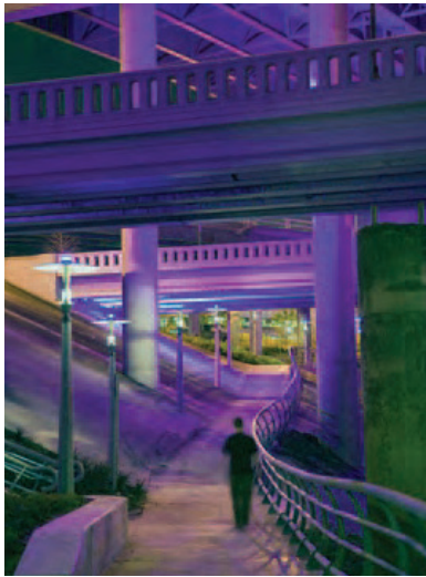
Figure 4.22 Highway underpass improvements
