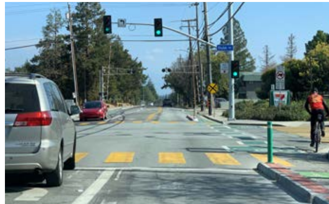
Figure 6.22 Examples of strategies recommended for Downtown's vehicular network: (far left) a high visibility crosswalk with a traffic circle, and (left) a protected left turn and separated bicycle path at a rail crossing.
