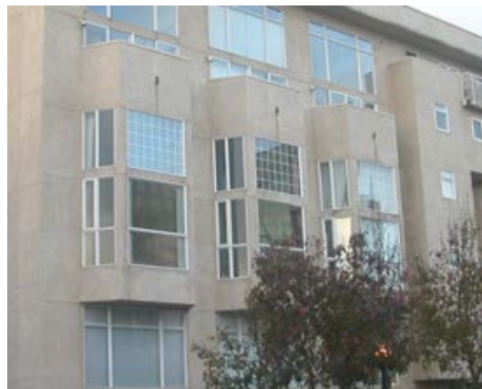
Example of Square Bay Window.
