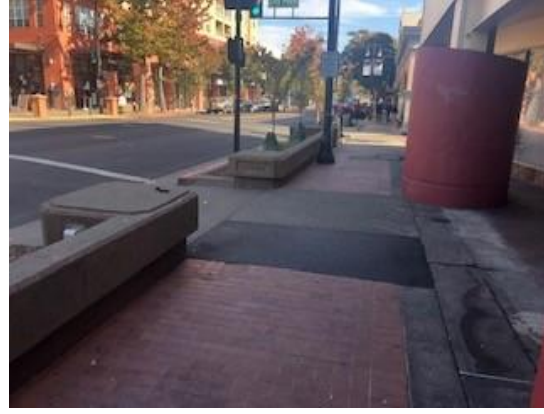
Current, built improvements at Fourth and Court Streets
