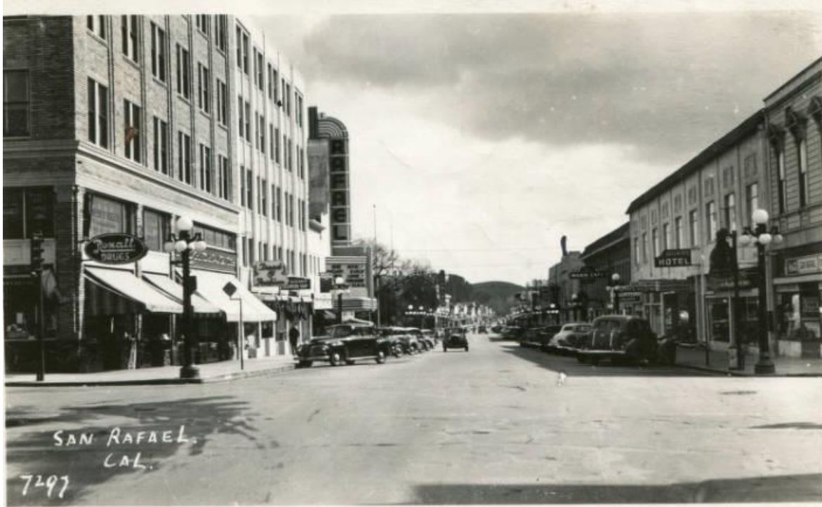
Postcard of San Rafael looking east down Fourth Street from B Street, circa 1947 (Marin County Free Library. Anne T. Kent California Room)
