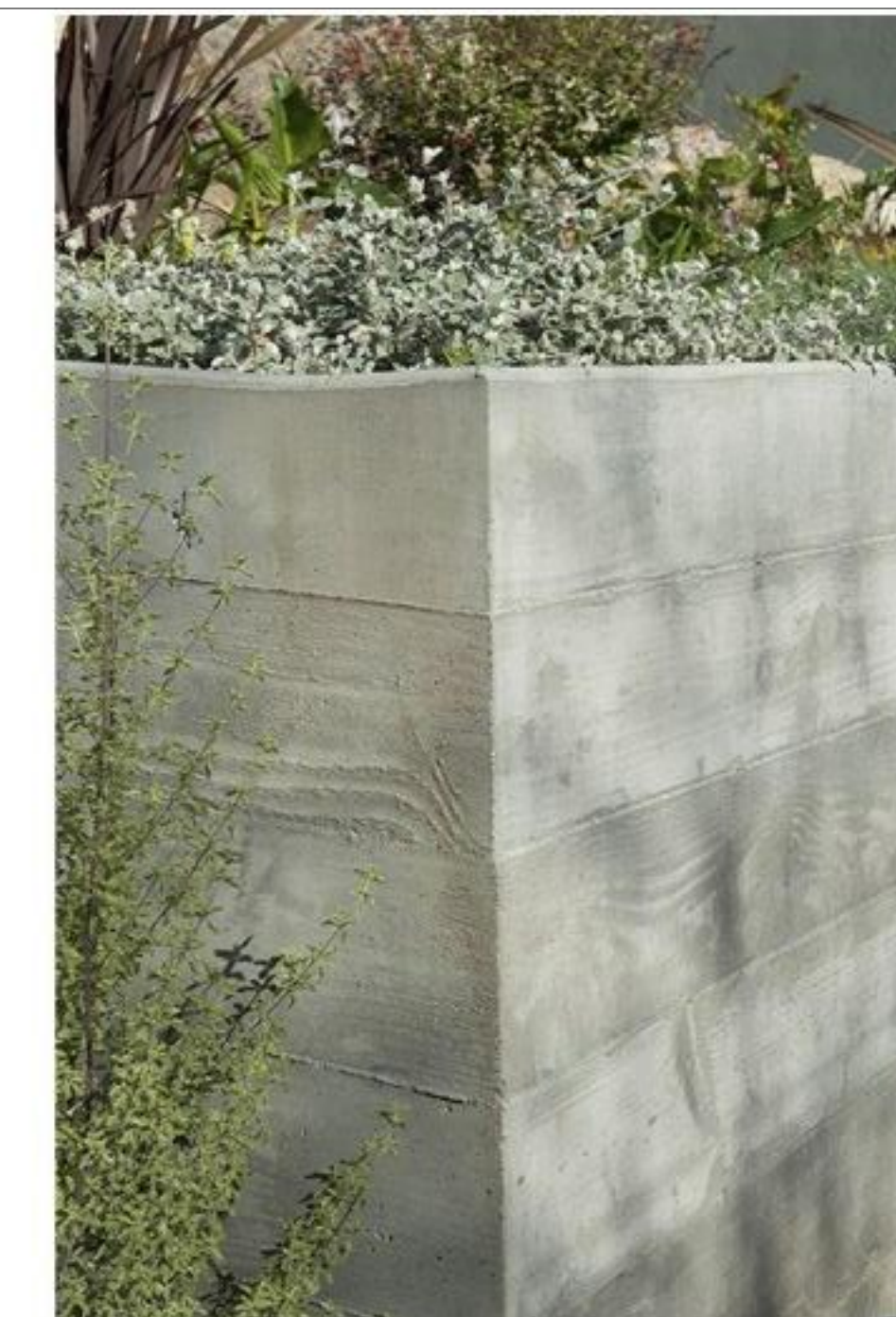
CONCRETE SITE WALLS
