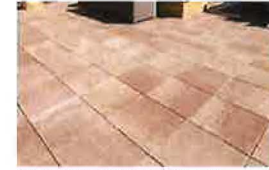
PEDESTAL PAVING SYSTEM- NEUTRAL COLORS TO COMPLIMENT THE MISSION STYLE OF THE ARCHITECTURE
