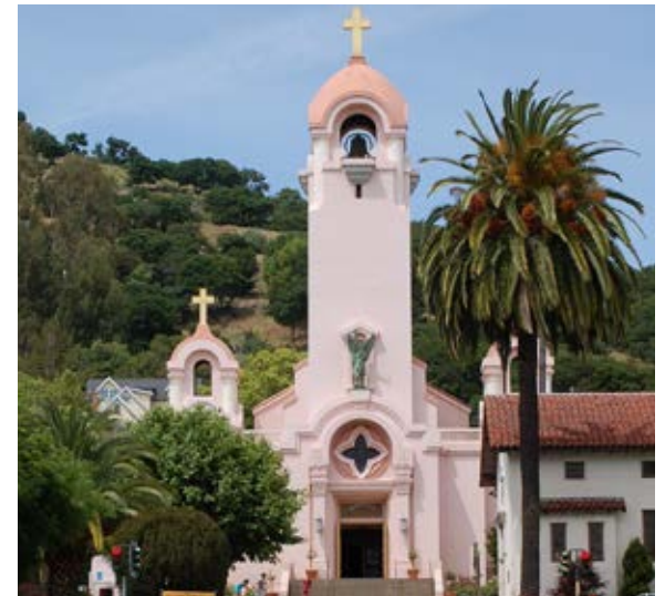
Figure 3.15 (Above) Existing historic and cultural resources in Downtown, such as the Boyd Gatehouse should be maintained and celebrated.
