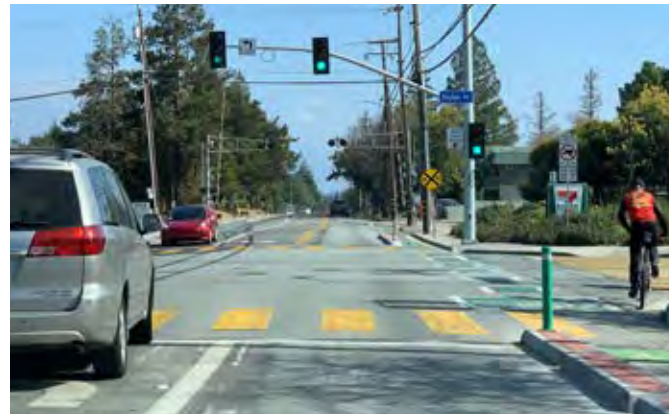
Figure 6.22 Examples of strategies recommended for Downtown's vehicular network: (far left) a high visibility crosswalk with a traffic circle, and (left) a protected left turn and separated bicycle path at a rail crossing.
