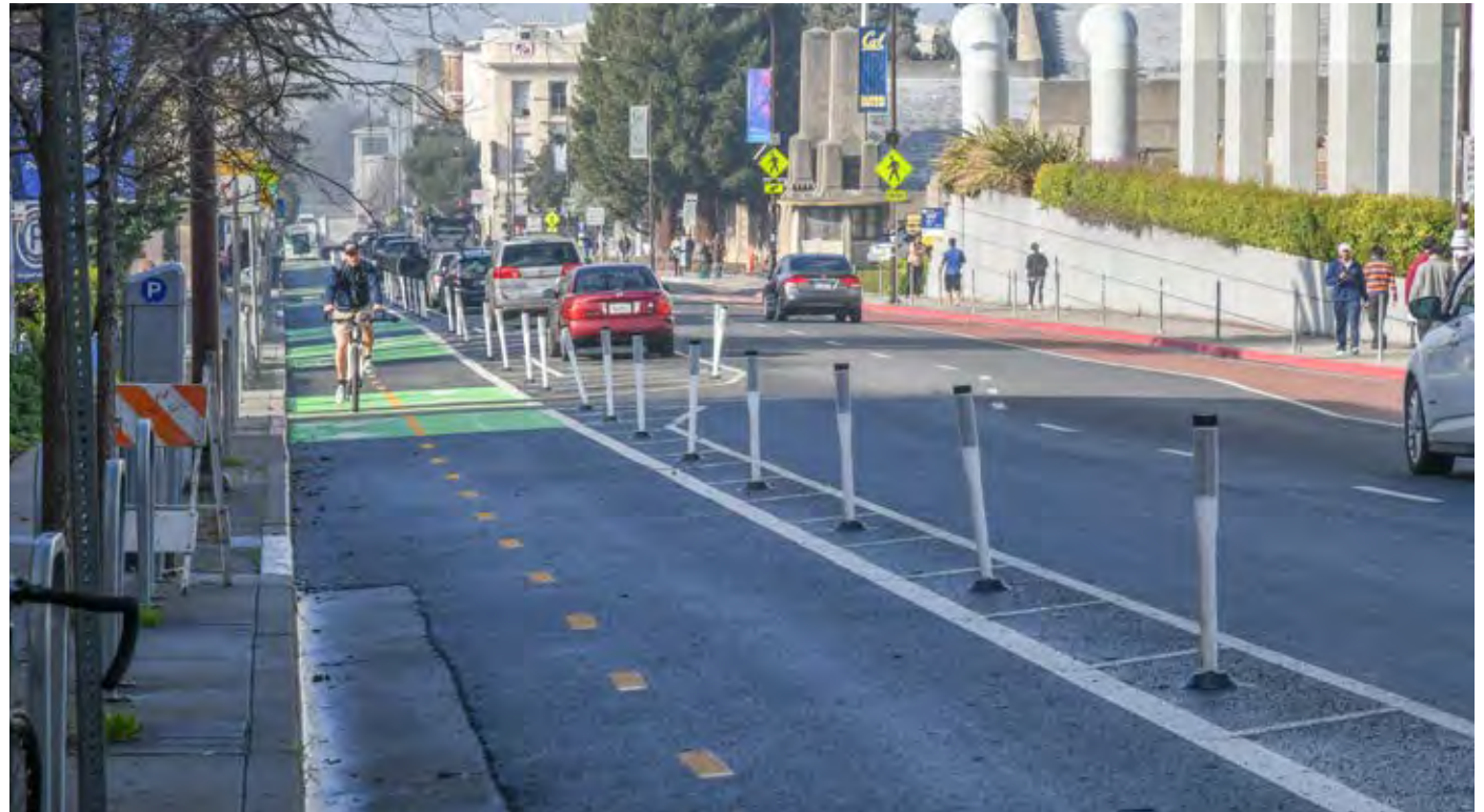
Figure 6.21 An example of a Complete Street: Bancroft Avenue, Berkeley, CA
