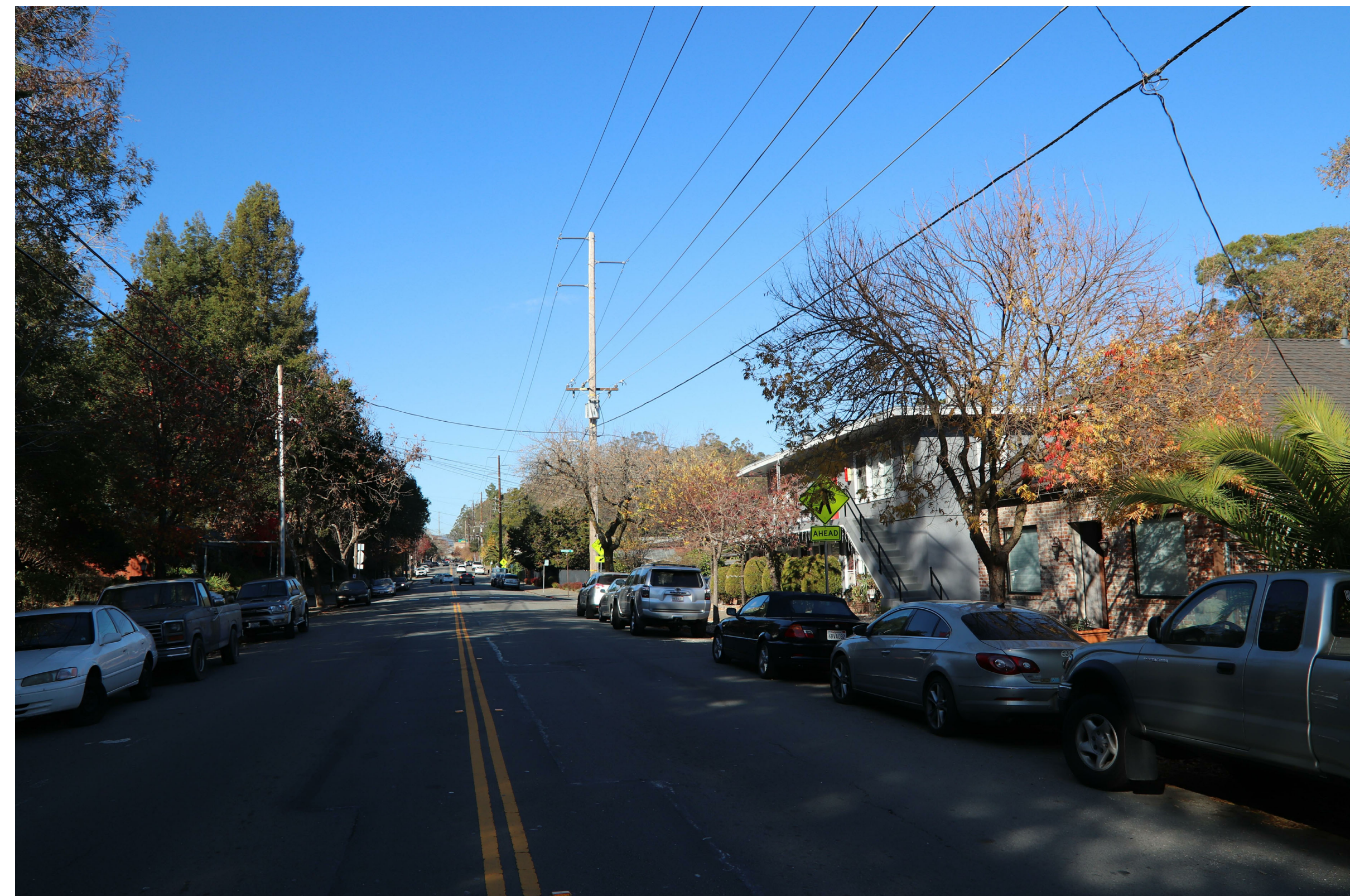
EXISTING NORTHBOUND LICOLN AVE VIEW
