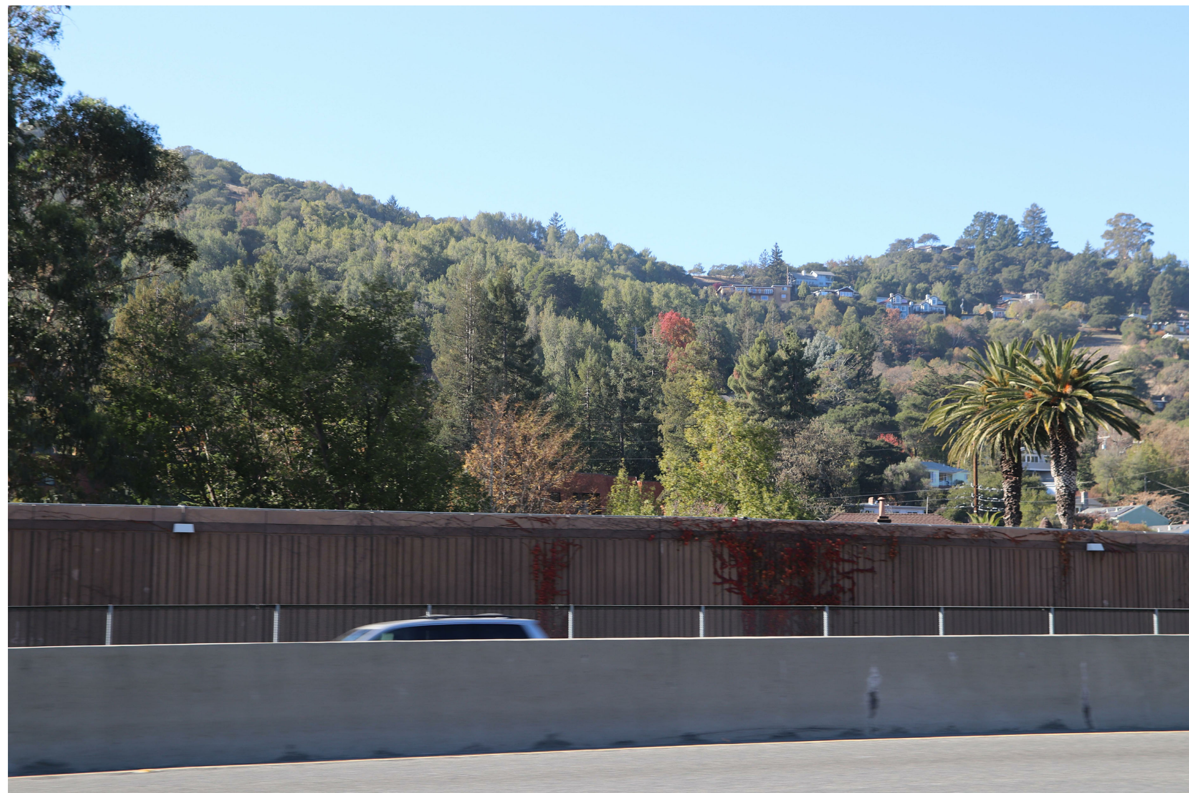
EXISTING NORTHBOUND FREEWAY VIEW
