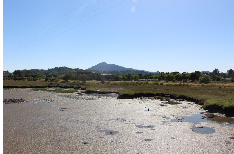
Photo 8 - View from the access ramp to the easternmost PG&E tower on the Project Site, looking toward the mudflat and eroded Tiscornia Marsh edge.
