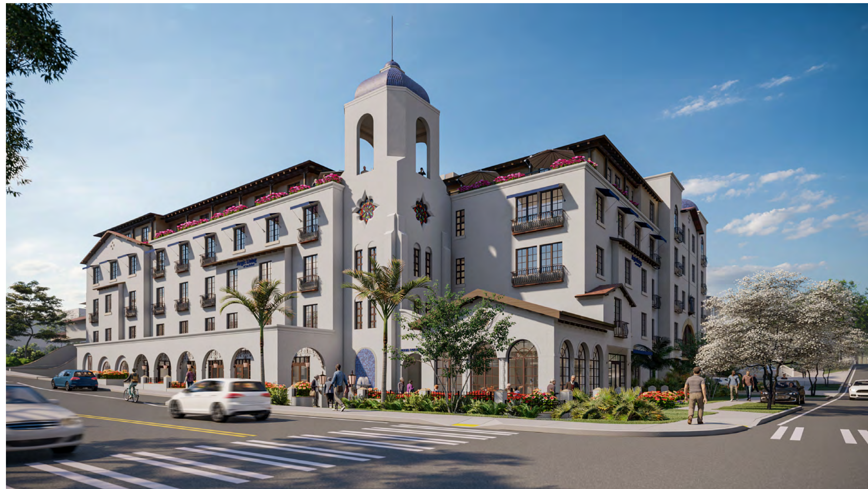
VIEW FROM INTERSECTION - MID DAY
