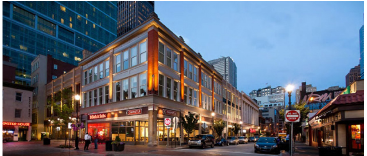
Figure 3.14 Renovation and adaptive use of historic buildings is sustainable and preserves a sense of history.
