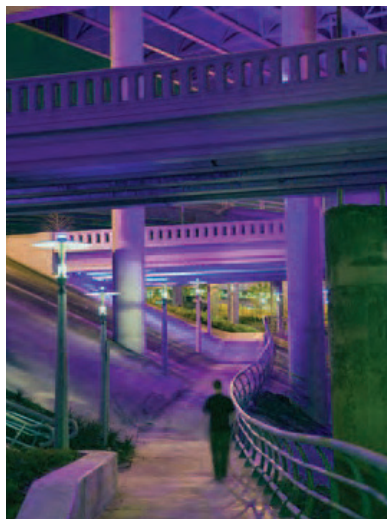
Figure 4.22 Highway underpass improvements
