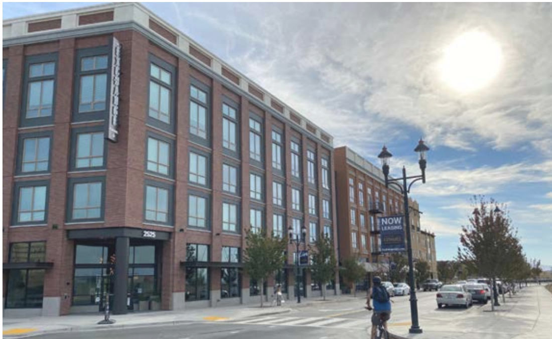
The top of the building is articulated with an entablature and parapet wall, Image source: www.719larkin.com
