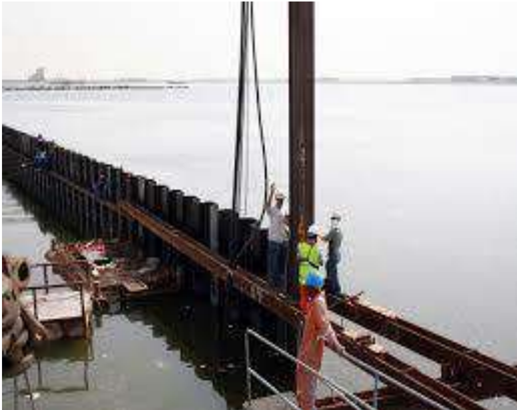
Tiscornia Marsh Habitat Restoration Aerial .D160888.0 Figure 27 Containment options: examples of bladder dam (top) and sheetpile wall (bottom).
