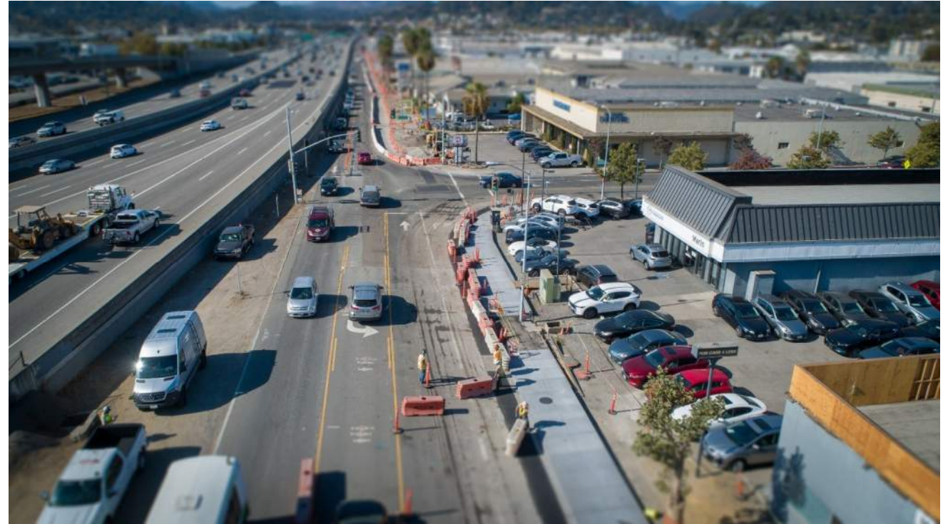
Francisco East Sidewalk Widening
