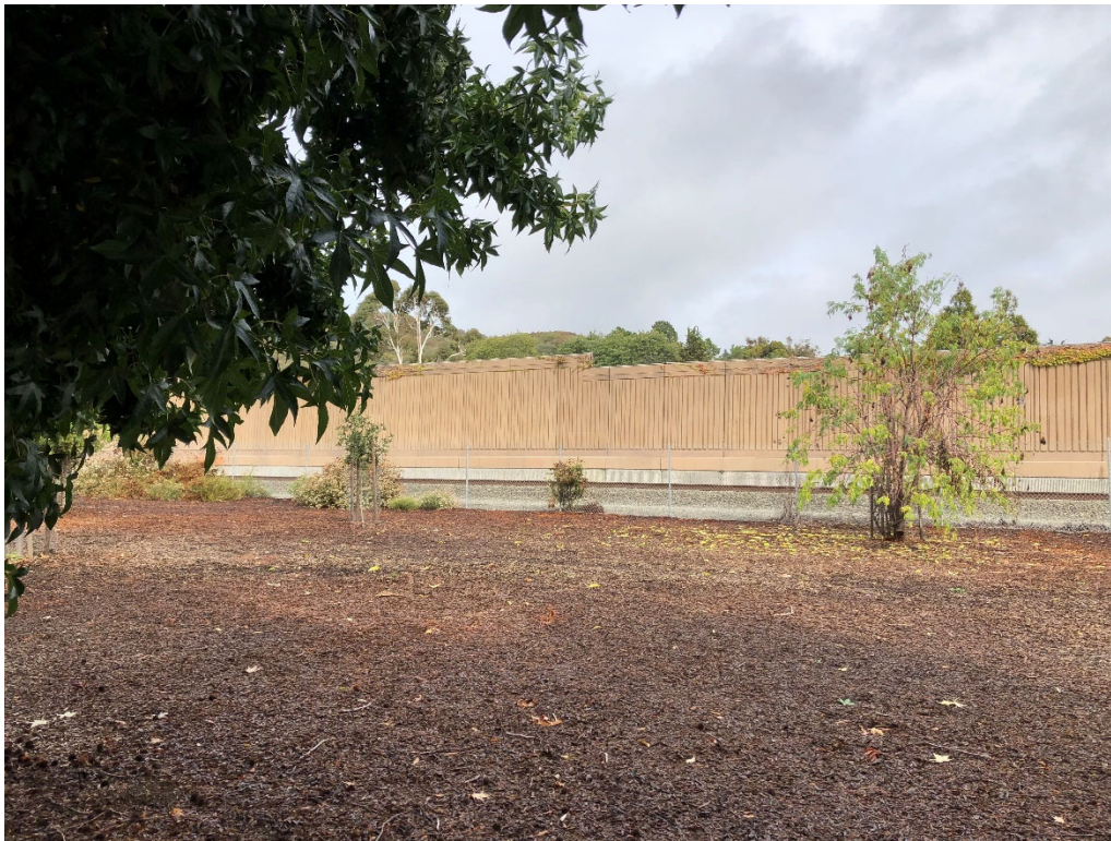
Photo 4. Railroad tracks and sound wall east of Brookdale Avenue (across the street from the project site).
