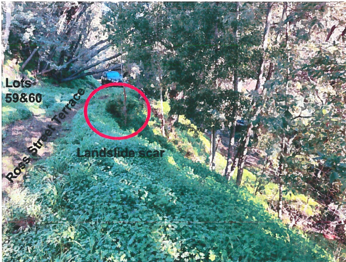
Figure 3. Evidence of a historic landslide located directly on the site. The landslide began at Ross Street Terrace and continued through 56 Clayton Street on to 64 Clayton Street.
