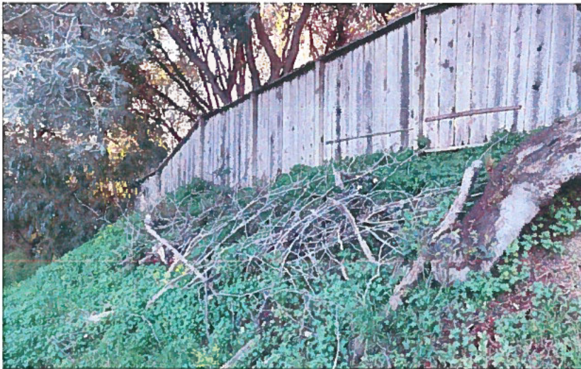
Figure 5. Vegetation dumped by the developer's contractor in July 2020. Pictured in November 2021.
