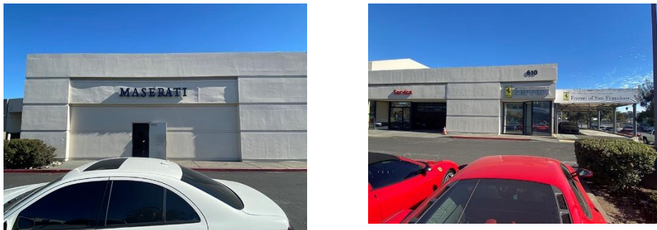
Image 2.4, 2.5 South Elevation (faces Du Bois Street) Building A
