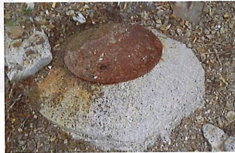
A non-corroded manhole on land.
