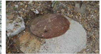
A non-corroded manhole on land.
