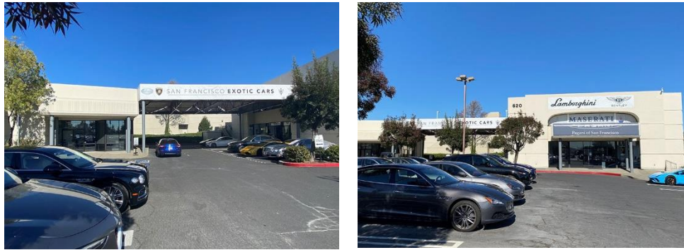
Image 2.6, 2.7 East Elevation (faces Rice Drive) Building A (left); canopy (center); Building B (right)
