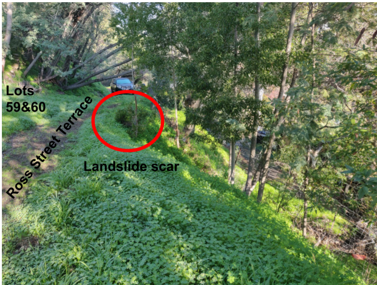
Figure 3. Evidence of a historic landslide located directly on the site. The landslide began at Ross Street Terrace and continued through 56 Clayton Street on to 64 Clayton Street.
