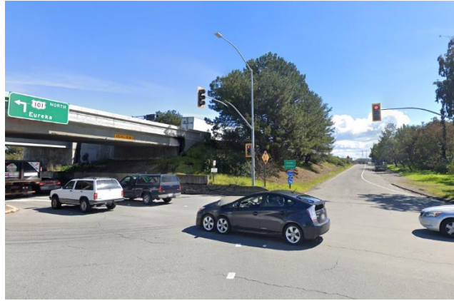
Bellam/I-580 west ramps (turning movement counts only) - 1 camera on the luminaire of the northwest corner.
