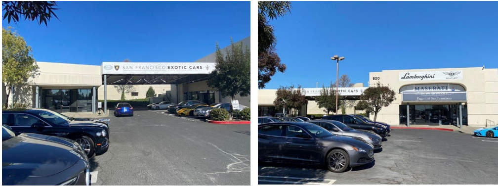
Figure 3.6, 3.7 East Elevation (faces Rice Drive) Building A (left); Service Canopy (center); Building B (right)
