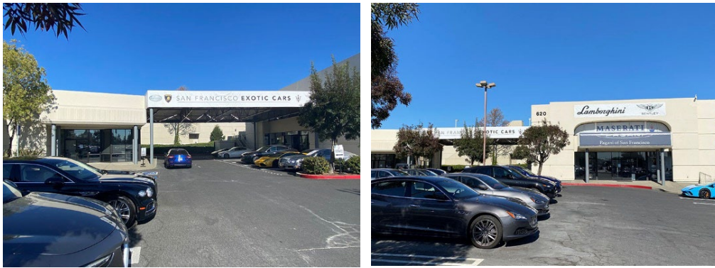
Figure 3.6, 3.7 East Elevation (faces Rice Drive) Building A (left); Service Canopy (center); Building B (right)
