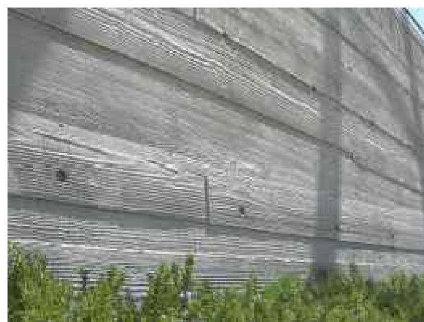
Poured concrete walls
