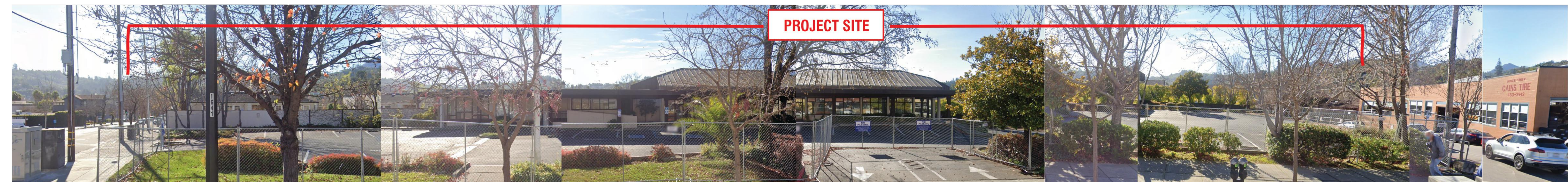
1. VIEW FROM 4TH STREET - SOUTH FACING
