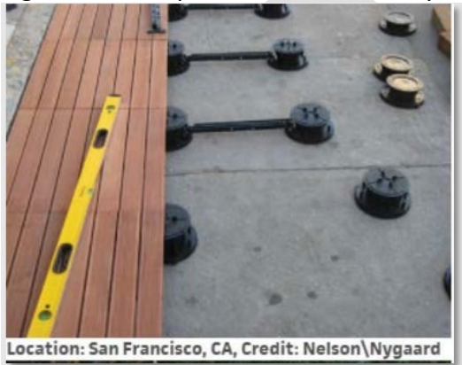
Figure 2: Bison pedestals for streetary sub-structure
