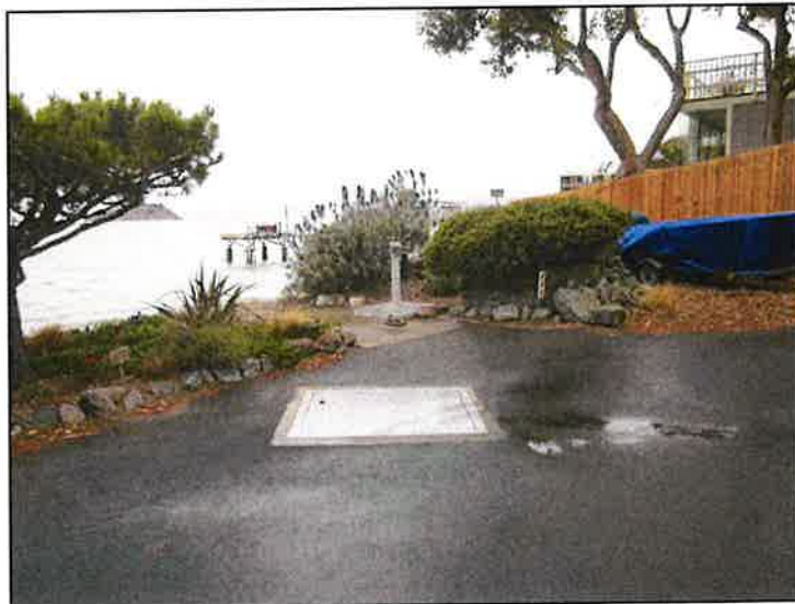
Beach Drive Pump Station
