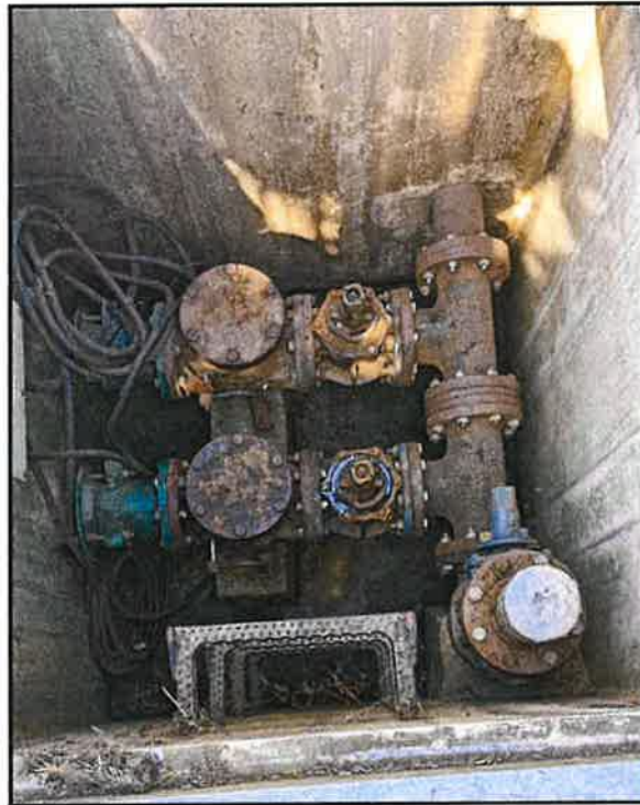
Beach Drive Pump Station Valve Pit
