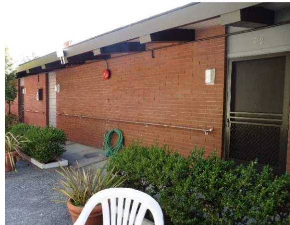
Figure 39. North façade, looking southeast.
