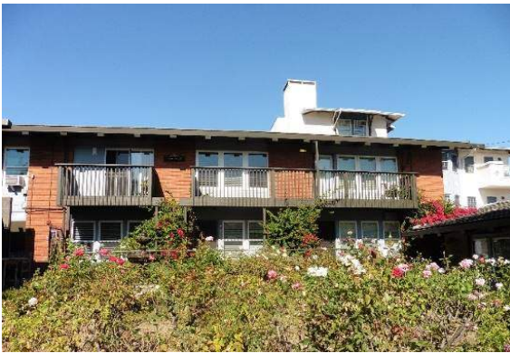
Figure 46. South façade, looking north.
