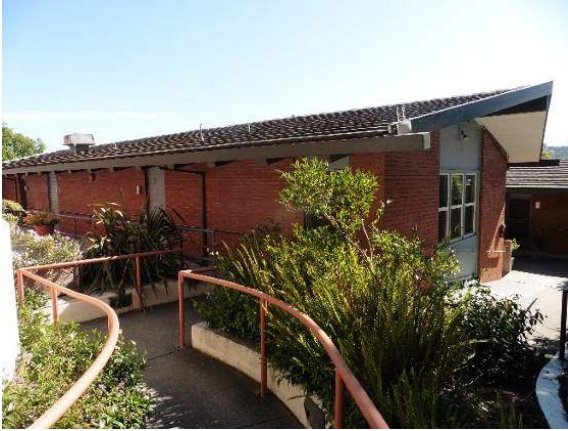
Figure 44. North and west façades, looking southeast.
