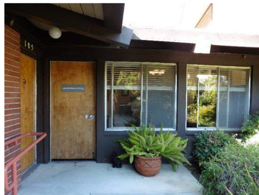
Figure 31. Single story left side of south façade.
