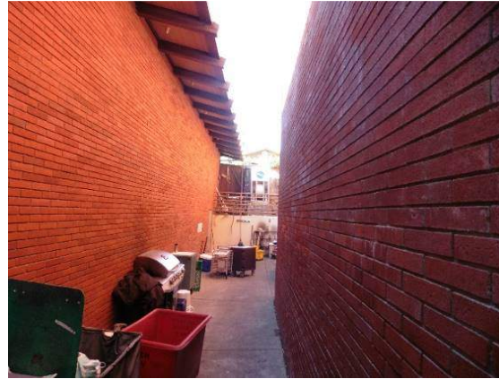
Figure 23. East façade and alleyway.
