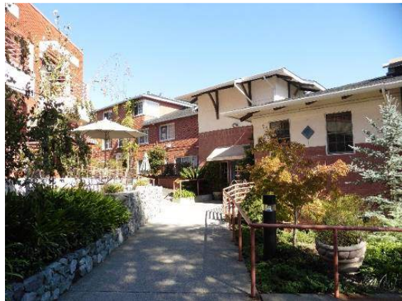
Figure 73. Concrete ramps to Assisted Living Facility, Minor Building, looking northeast.
