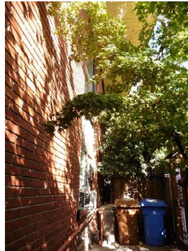
Figure 29. South façade of long leg, looking east.
