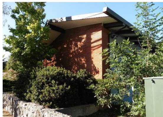
Figure 43. South façade, looking southwest.
