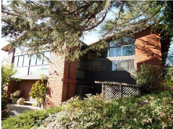
Figure 22. South façade, looking north.
