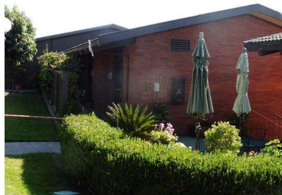
Figure 25. Northern section, north façade, looking south.
