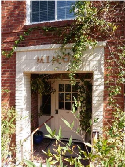
Figure 58. Close-up view of the recessed main entry, looking east.
