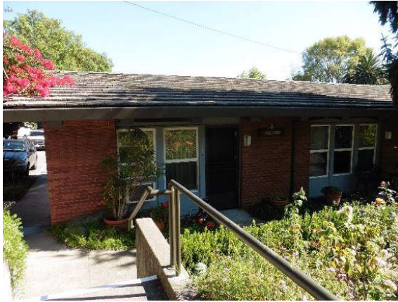
Figure 40. West façade, looking east.
