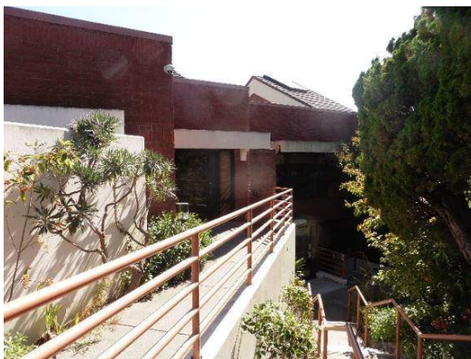
Figure 64. Eastern section of the north façade, looking southwest.
