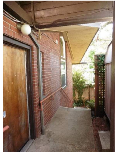
Figure 27. North façade (right side) and utility door, looking west towards stairway.
