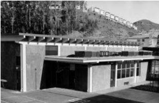
Figure 131. Clarendon Elementary School, Wurster, Bernardi, and Emmons, 1960. Source: San Francisco Public Library.
