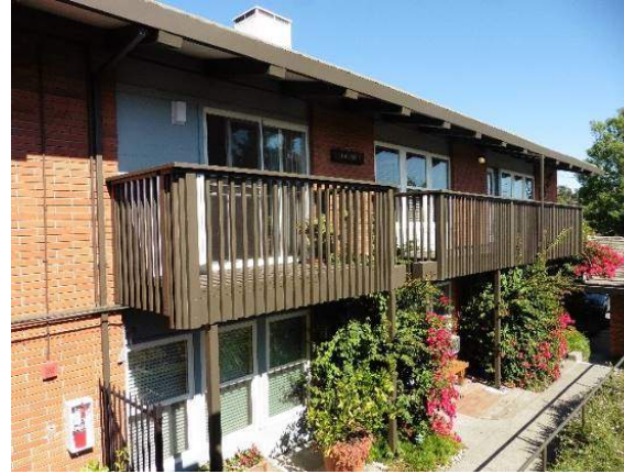
Figure 45. South façade, looking northeast.
