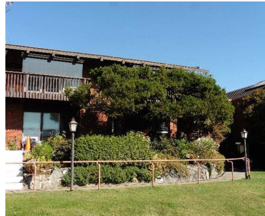
Figure 13. West façade (right side), looking east.
