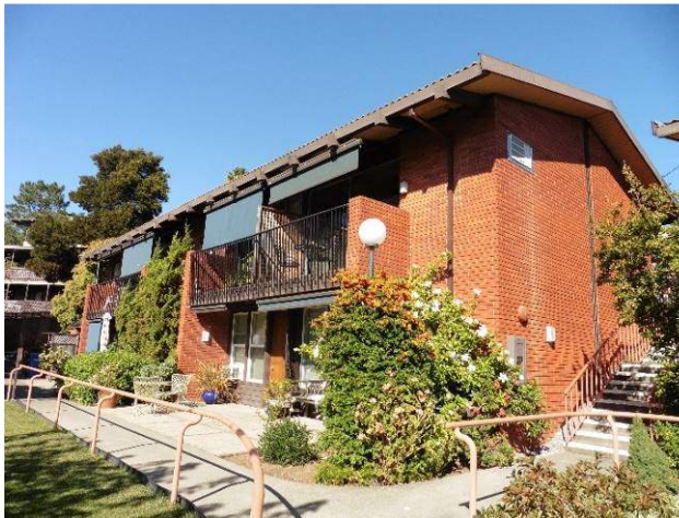
Figure 16. West façade, viewed facing northeast.
