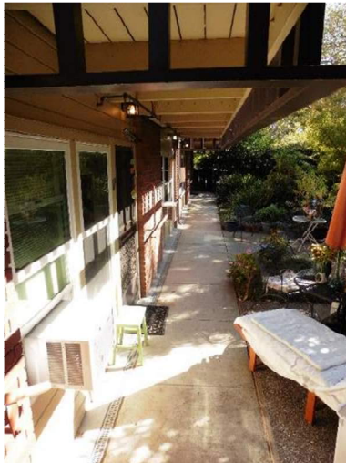
Figure 28. West façade ground story, looking south below balcony.
