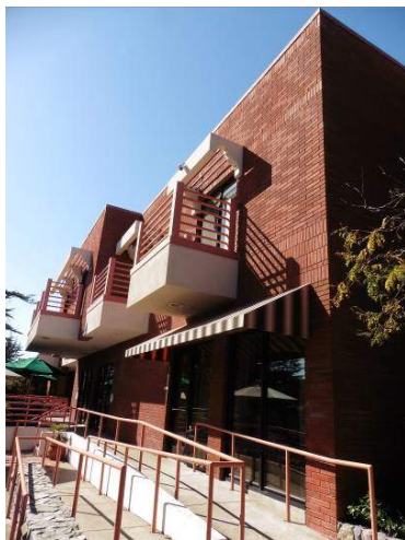
Figure 62. East side of the south façade, looking northwest.
