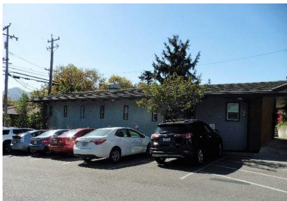
Figure 42. East façade, looking southwest.
