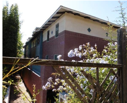
Figure 53. East façade (northern section) and rear façade, looking south.
