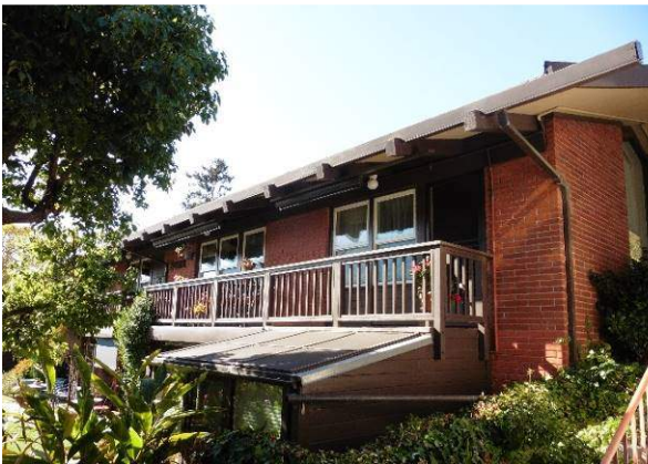
Figure 34. Second story of south façade.
