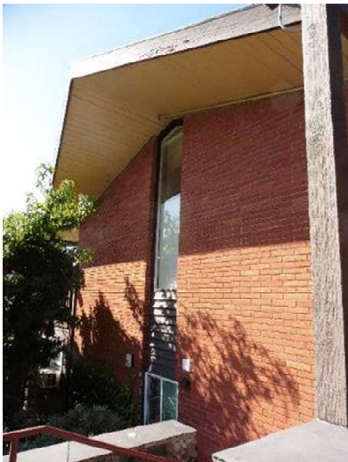
Figure 4. South façade, looking northwest.
