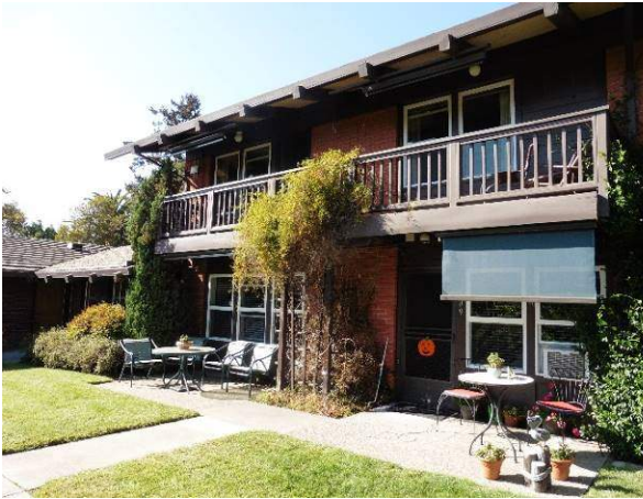
Figure 32. Two-story portion of south façade (left side), looking northwest.
