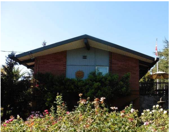
Figure 38. East façade, looking west.
