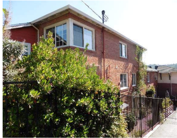
Figure 55. Three-story portion of northwest corner and west façade, looking south.
