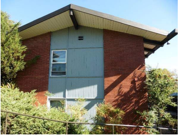
Figure 36. West façade, looking east.
