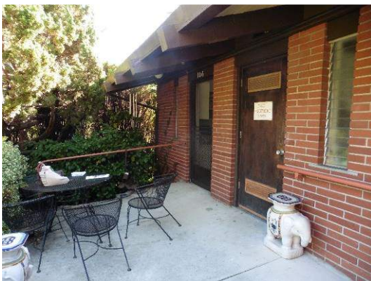
Figure 30. East façade of short leg, looking south.
