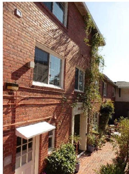
Figure 57. West façade, looking towards entries and two-story portion (southern section).
