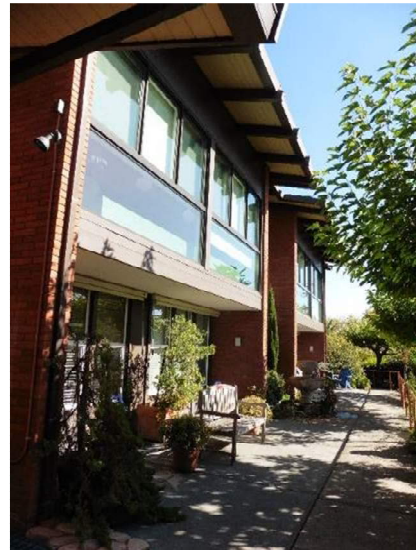
Figure 21. Southern section, west façade.
