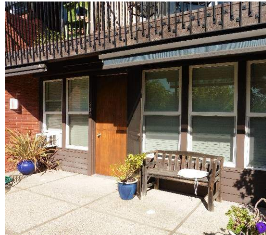
Figure 17. Close-up view of west façade unit entry, looking northeast.
