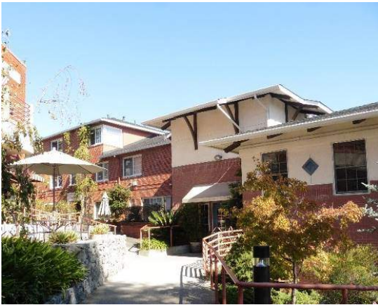
Figure 48. West façade at connection, looking northeast.
