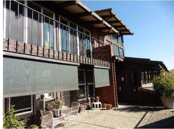
Figure 19. Close-up view of west façade towards entry bay, looking southeast.
