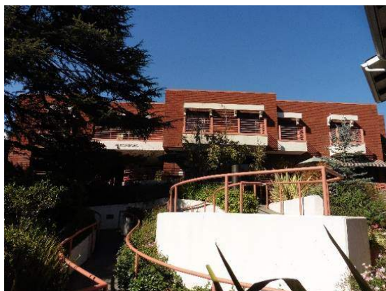
Figure 83. Ramps leading up to Skilled Nursing Building, looking north.
