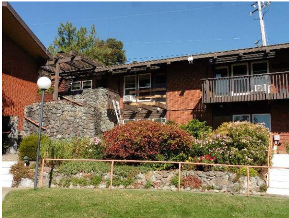
Figure 12. West façade (left side), looking east.
