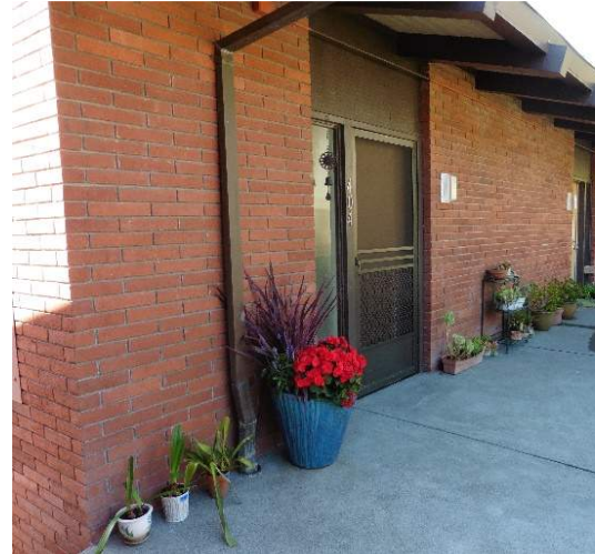
Figure 15. East façade, looking north.
