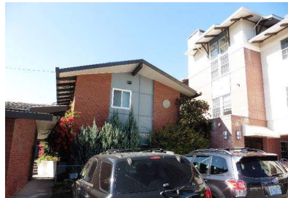
Figure 47. East façade, looking west.
