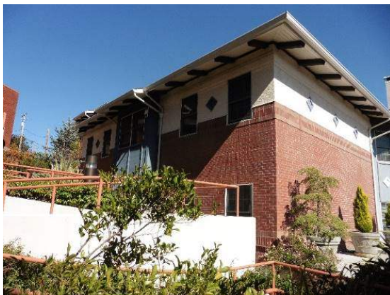
Figure 50. West façade (southern section) and south façade (western section).
