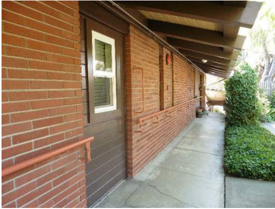
Figure 26. North façade (left side), looking west.
