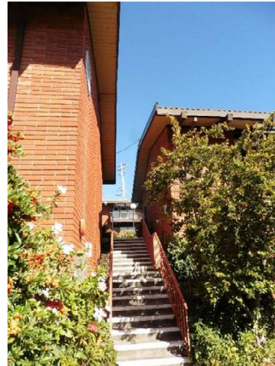
Figure 86. Concrete stairs connecting campus levels, stairway between Buildings C and D shown, looking east.
