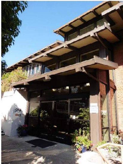
Figure 20. Entry bay of southern section.
