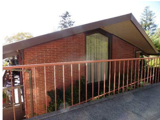
Figure 35. East façade of long leg, looking west.
