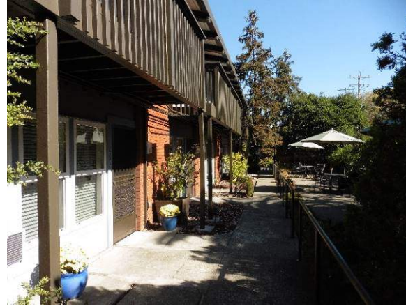
Figure 37. South façade, looking east.
