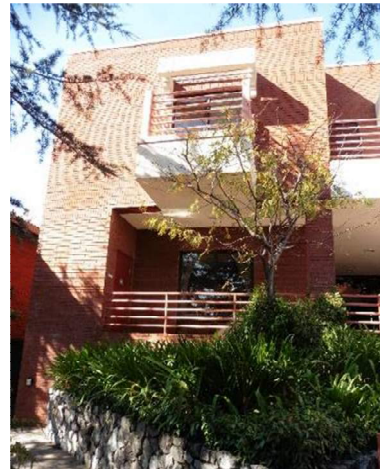
Figure 61. West side of the south façade, looking north.
