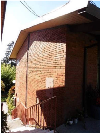
Figure 14. South façade, looking northwest.
