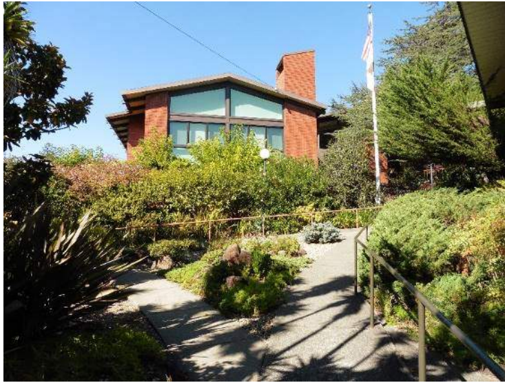
Figure 66. Pathways leading to Main Stair, looking north toward Administration Building.
