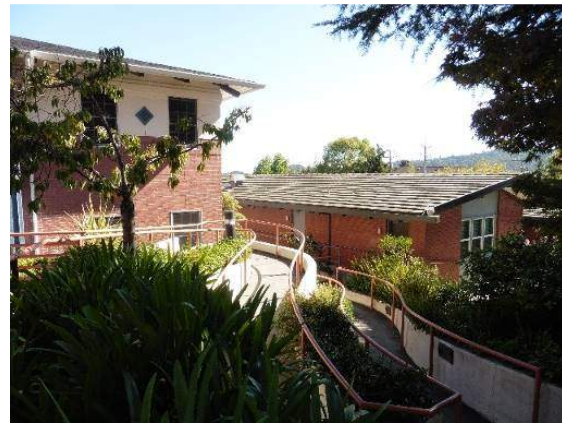
Figure 74. Ramps to Assisted Living Facility and Rose Garden residences, looking southeast.
