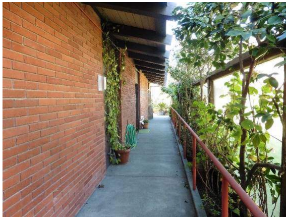
Figure 24. Northern section, east façade, looking north.
