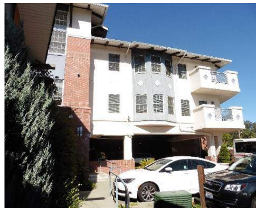
Figure 51. South façade (eastern section).
