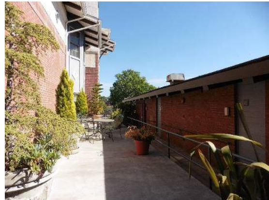
Figure 76. Concrete patio outside south façade of Assisted Living Facility, looking east.
