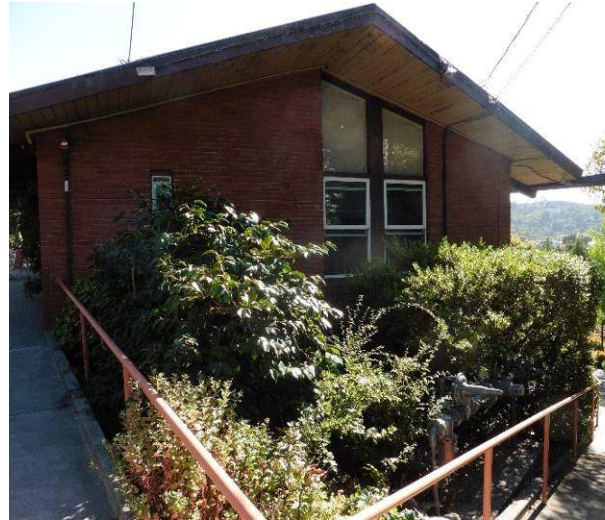
Figure 7. North façade, looking southwest.
