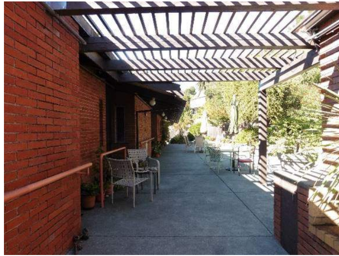
Figure 5. East façade and trellis, looking north.
