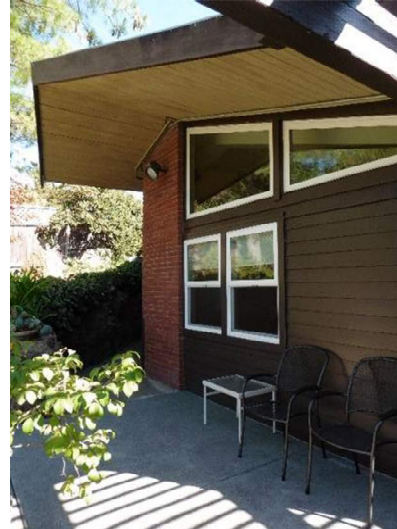
Figure 11. North façade, looking east.
