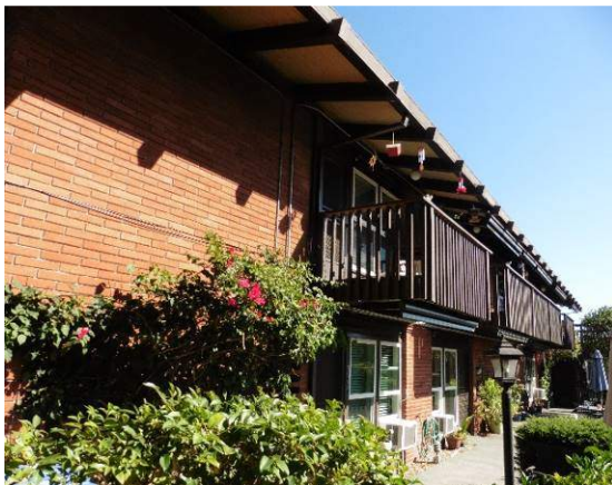
Figure 8. West façade, looking south.
