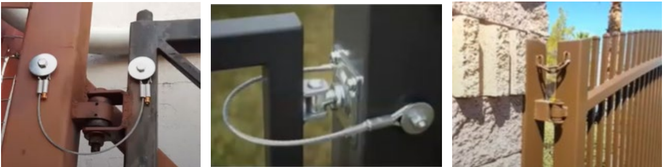
Figure 1. Examples of Swing Gate Fall-Over Protection
