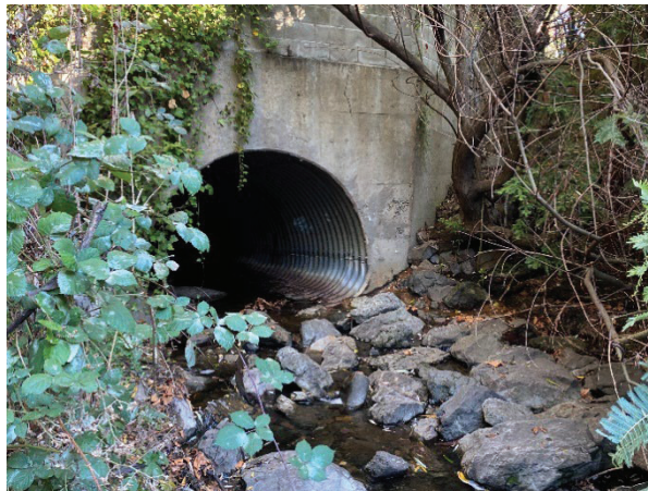
View of the endwall and open channel downstream of the CMP culvert.
