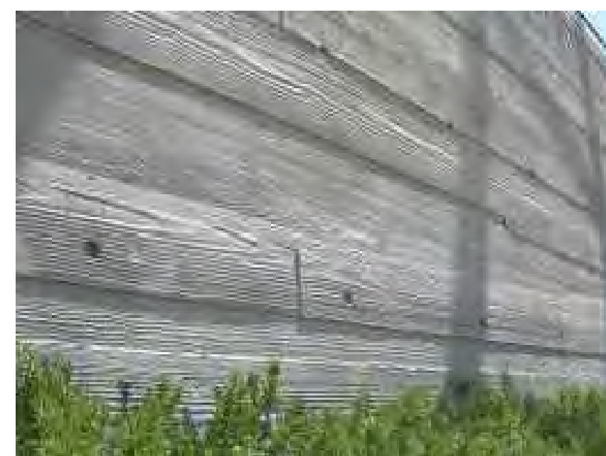
Poured concrete walls
