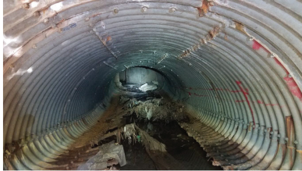
Upstream view of the arch CMP culvert showing the corroded floor and bowed flow line.
