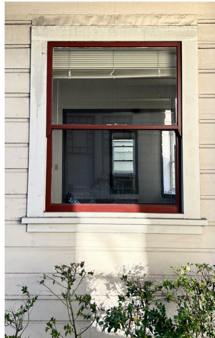
Photo 4: Subject window, November 2022
