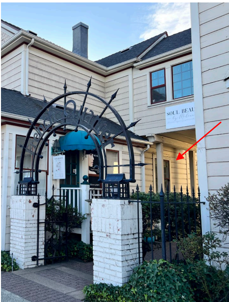
Photo 3: Subject window view from public street (looking southwest), November 2022
