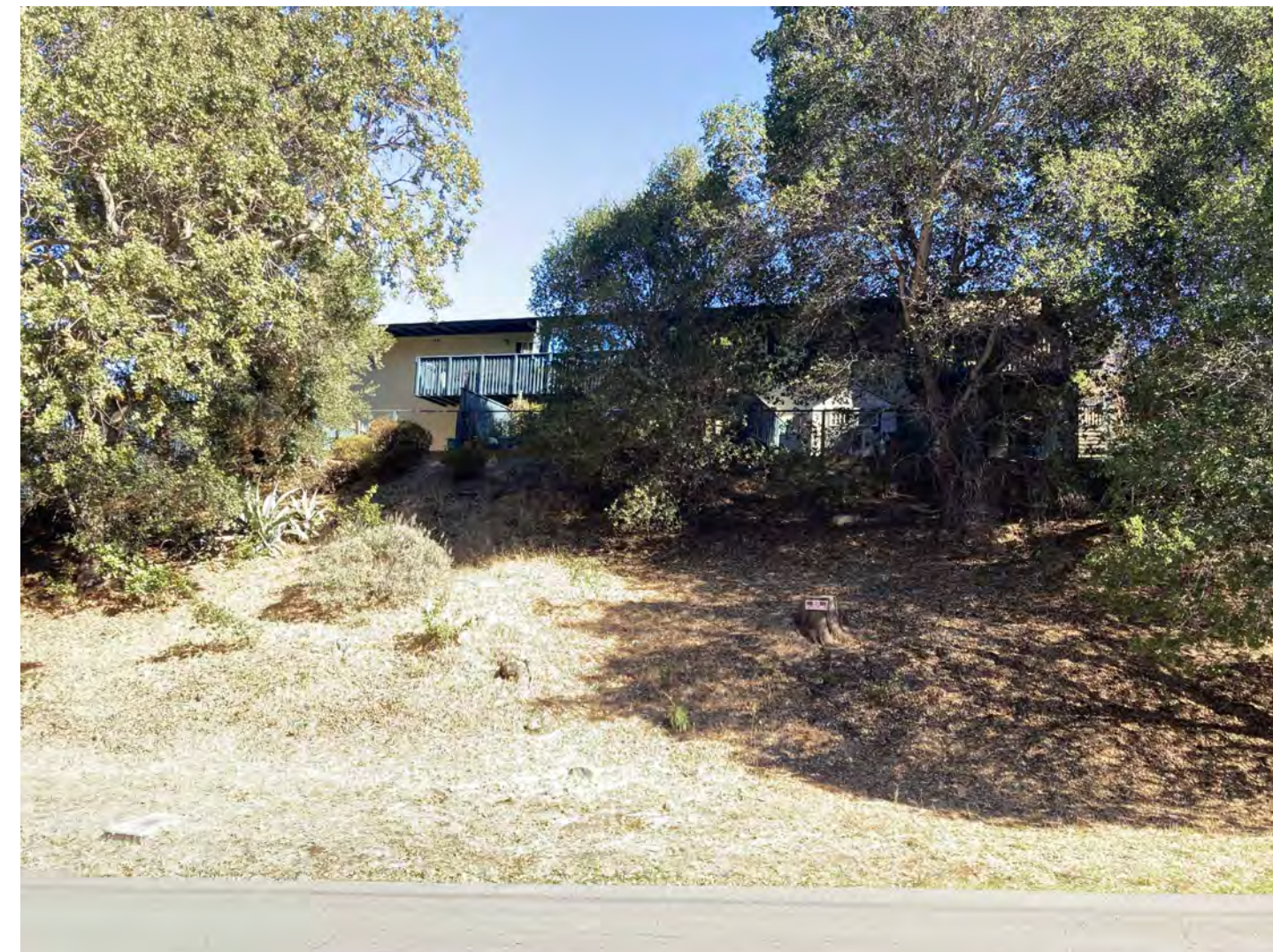
#7 - VIEW AT FRONT OF EXISTING 50 MERRYDALE APARTMENT BUILDING - FACING EAST
