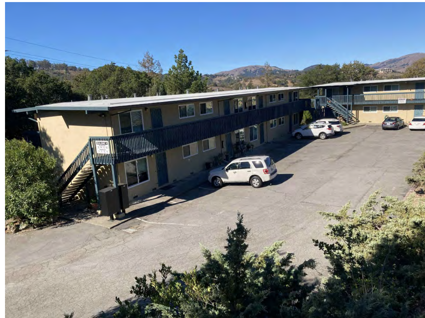
#8 - VIEW AT SIDE OF EXISTING 50 MERRYDALE APARTMENT BUILDING - FACING NORTH FROM SUBJECT SITE
