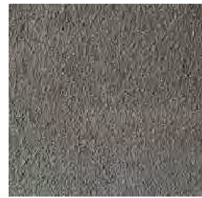
③ 3-COAT STUCCO SIDING, LAHABRA SAND FINISH COLOR: "WARM GRAY"
