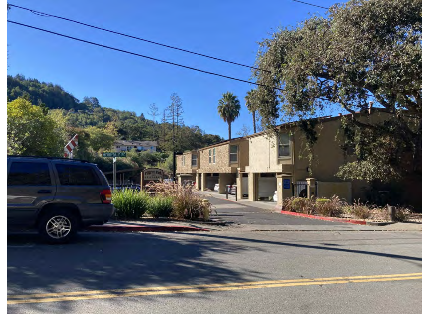
#11 - FACING NORTHWEST FROM MERRYDALE - NEIGHBORING BUILDINGS ALONG WEST SIDE OF MERRYDALE (ACROSS FROM SUBJECT SITE)
