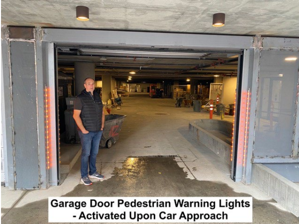
Exhibit 1: Flashing Light System
