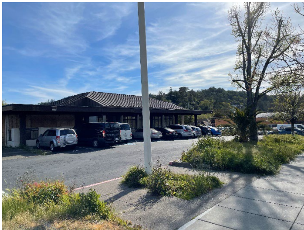
The current building at 1515 4 th St.
