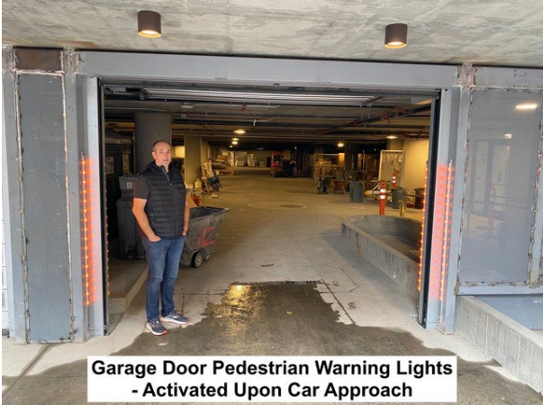
Exhibit 1: Flashing Light System
