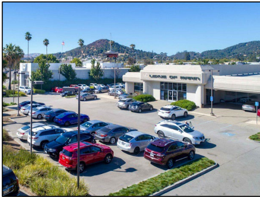
Figure 4: Existing South (Front) Elevation (looking northeast)
