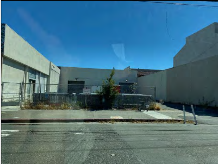
Photograph 1: View of the subject property facing south.
