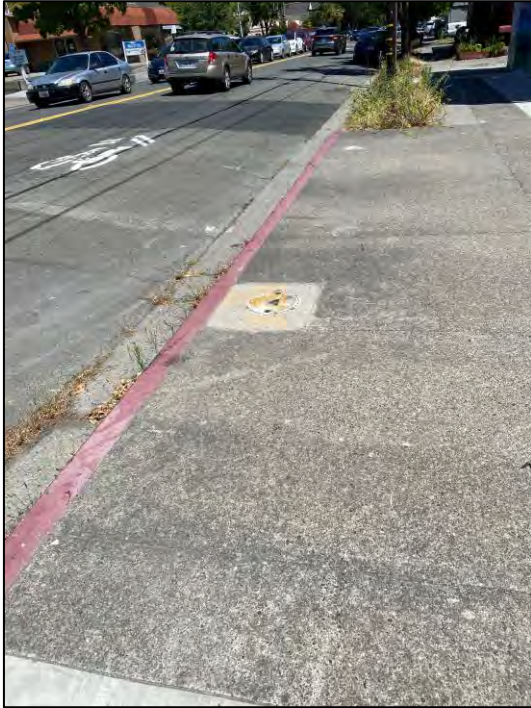
Photograph 17: Monitoring well located in sidewalk to the north of the subject property.
