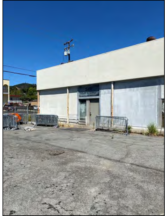
Photograph 2: Eastern portion of the building used for fire department storage.
