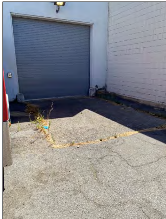
Photograph 4: Southwest corner of the building and location of former waste oil UST.
