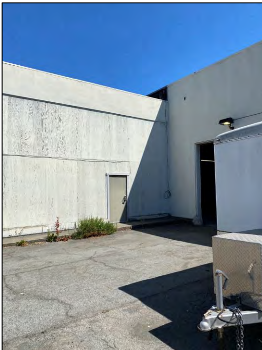
Photograph 3: Southeast corner of the building.
