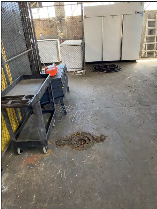
Photograph 11: Hydraulic lift in eastern portion of subject building, currently used for police evidence storage.
