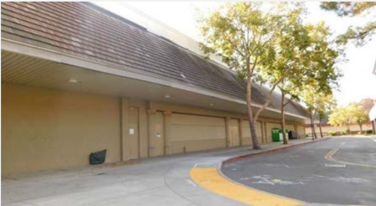
Photograph 8. Northgate Mall Unit 4: West (main) elevation, view to southeast (DSCN9420)
