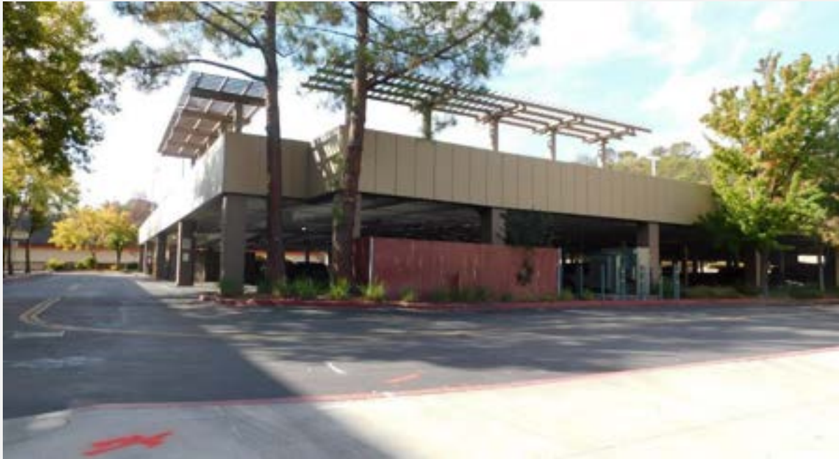
Exhibit 32. Parking Garage: West and north elevations, view to southwest (DSCN9423)
