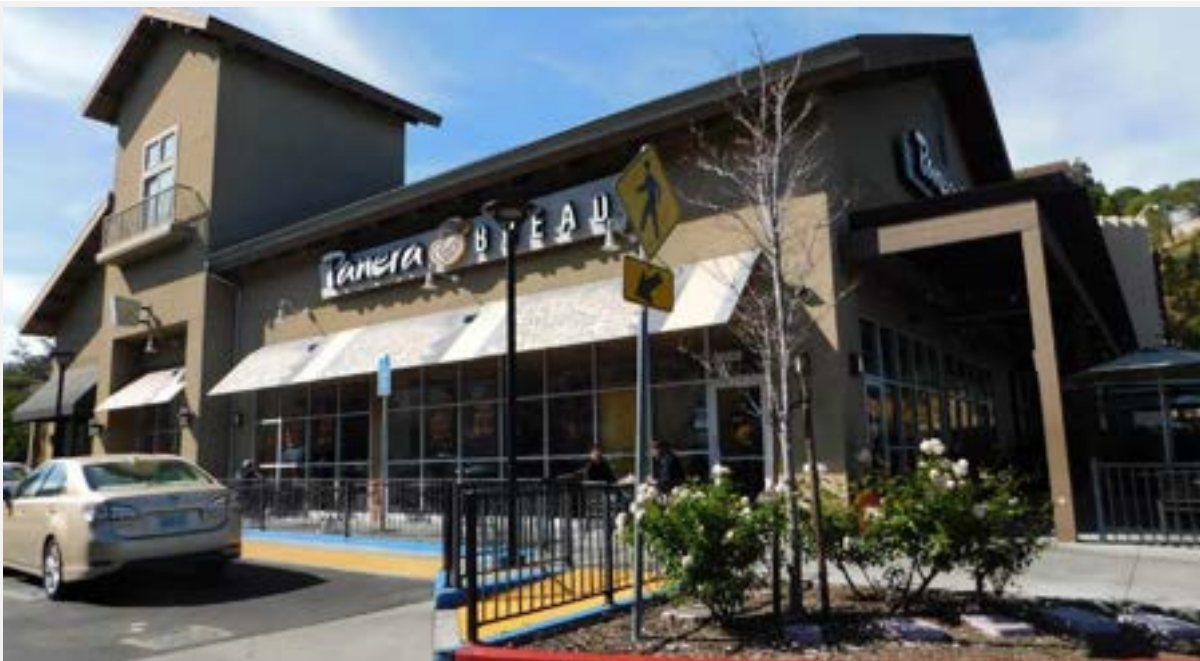
Photograph 21. Panera: South and west elevations, view to northwest (DSCN9562)
