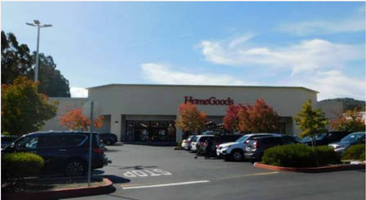
Photograph 19. Home Goods: West and north elevations, view to southwest (DSCN9533)
