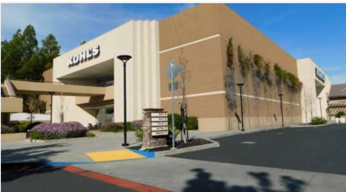
Photograph 17. Kohl's: South and West (main) elevations, view to northwest (DSCN9559)
