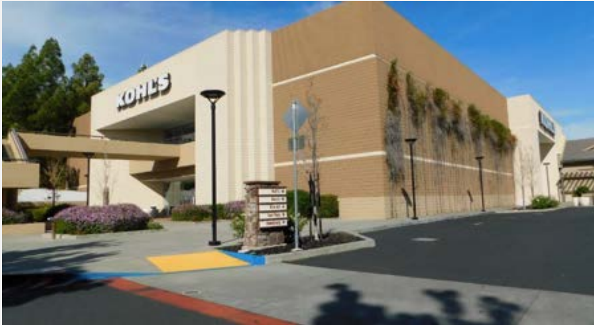
Exhibit 31. Kohl's: South and West (main) elevations, view to northwest (DSCN9559)
