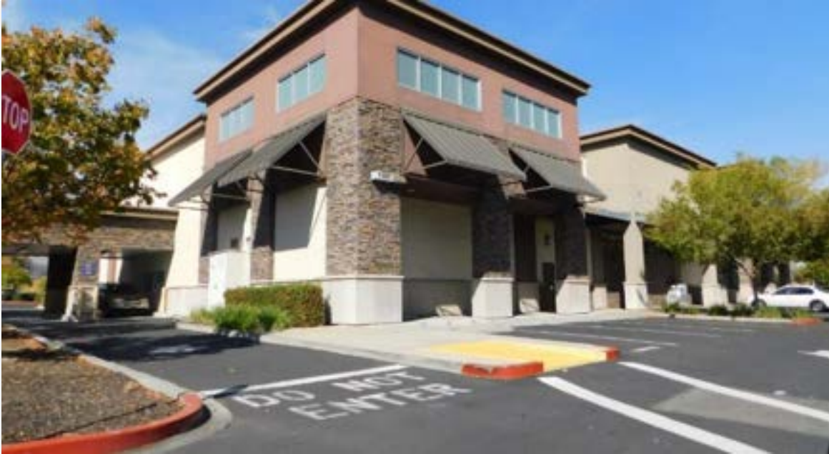
Exhibit 34. Rite Aid: South and west elevations, view to northwest (DSCN9545)
