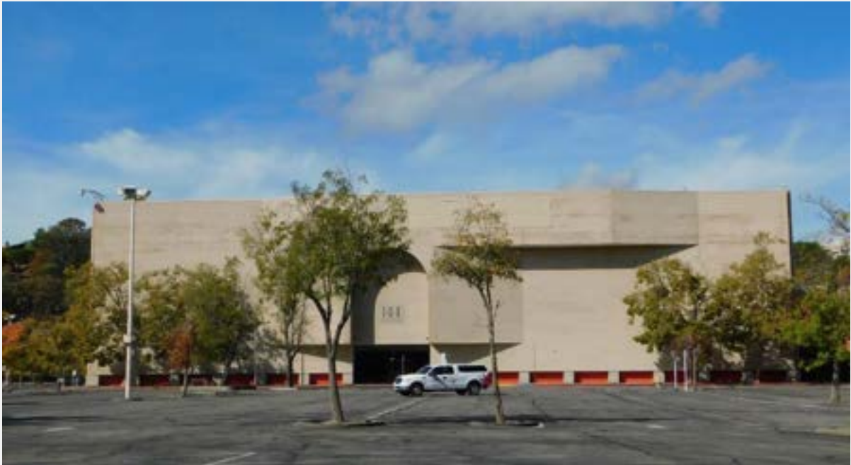
Photograph 12. Sears: East elevation, view to west (DSCN9502)
