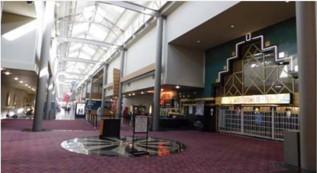
Photograph 10. Northgate Mall Unit 4 and 5: Now enclosed space between Units 4 and 5, view to north (DSCN9443)
