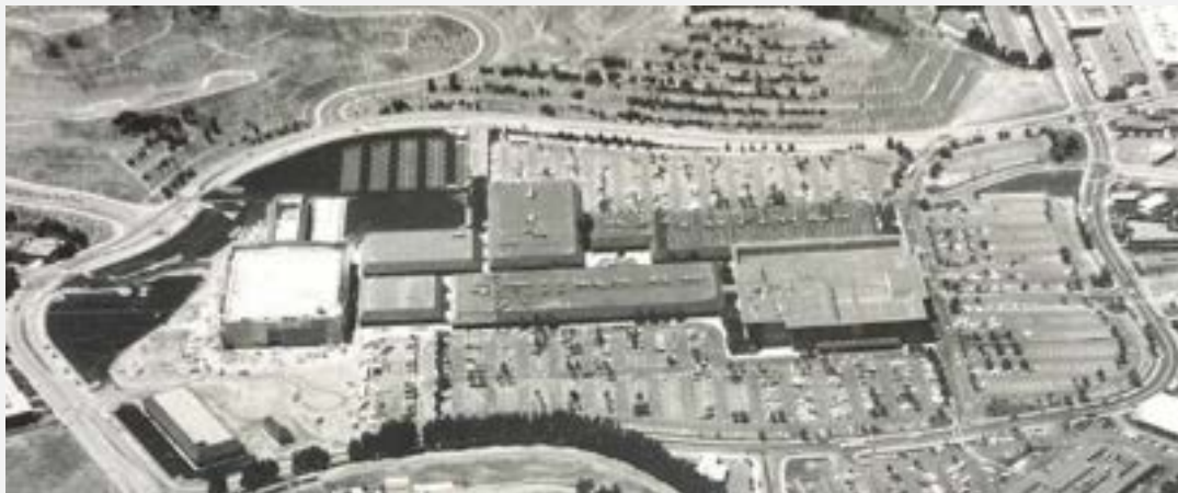
Exhibit 10. Detail of a historical aerial photograph in 1972 showing Units 4 and 5 between the nearly completed Sears buildings at the far left and the original 1964 sections of the Northgate Mall at right (Courtesy of the Marin History Museum Brady Collection)
