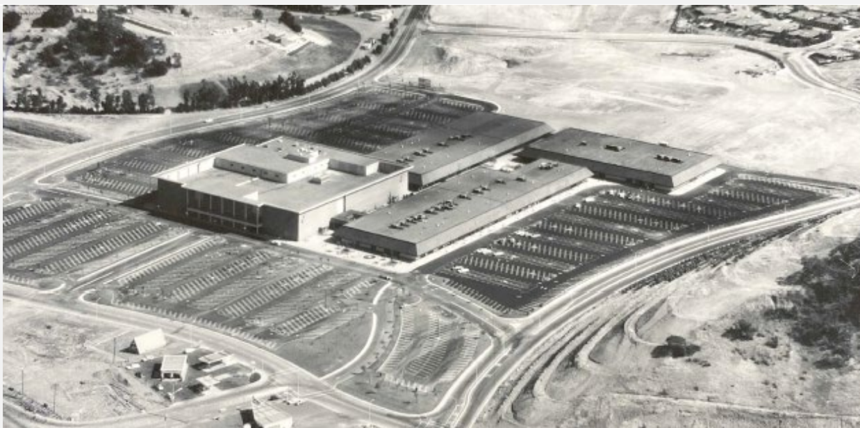
Photograph 26. Detail of a historical aerial photograph looking southwest at the Northgate Mall as it appeared in 1965 with the Emporium building at the left foreground flanked by Northgate Mall Units 1, 2, and 3. (Courtesy of the Marin History Museum Brady Collection)
