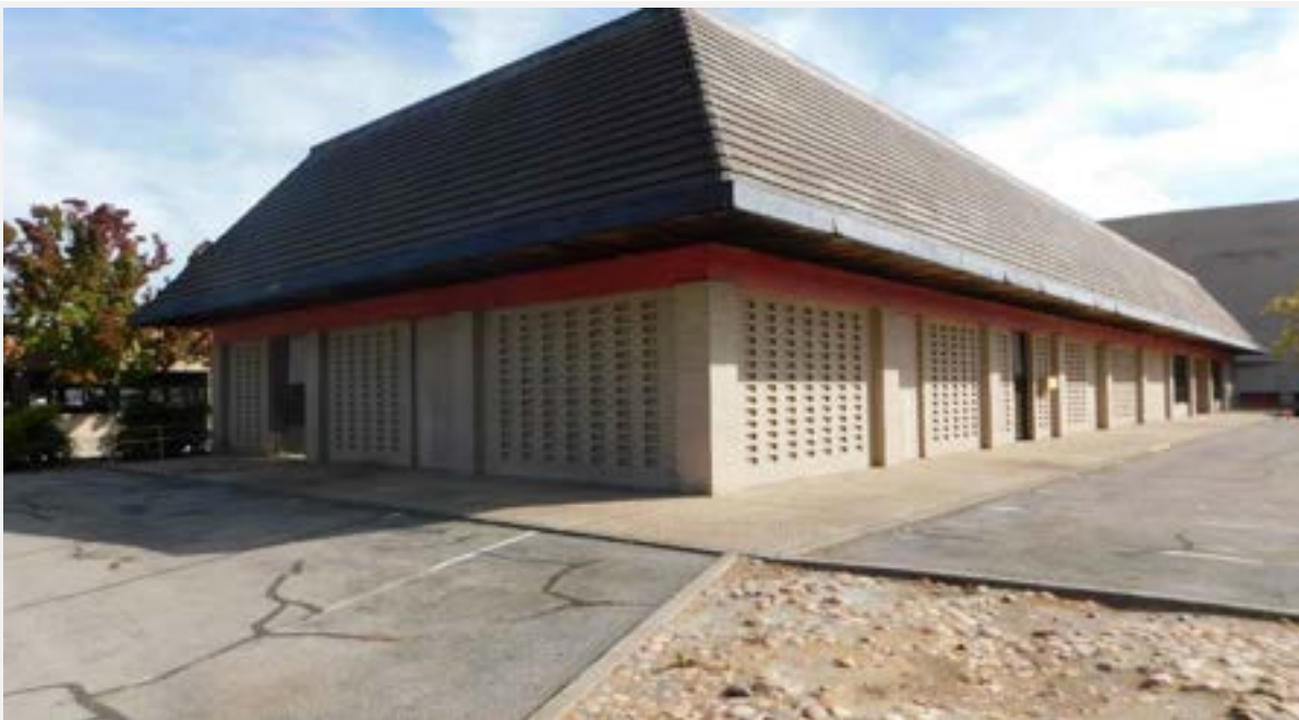
Photograph 15. Sears Seasonal Sales Building: West and south (main) elevations, view to northeast (DSCN9454)
