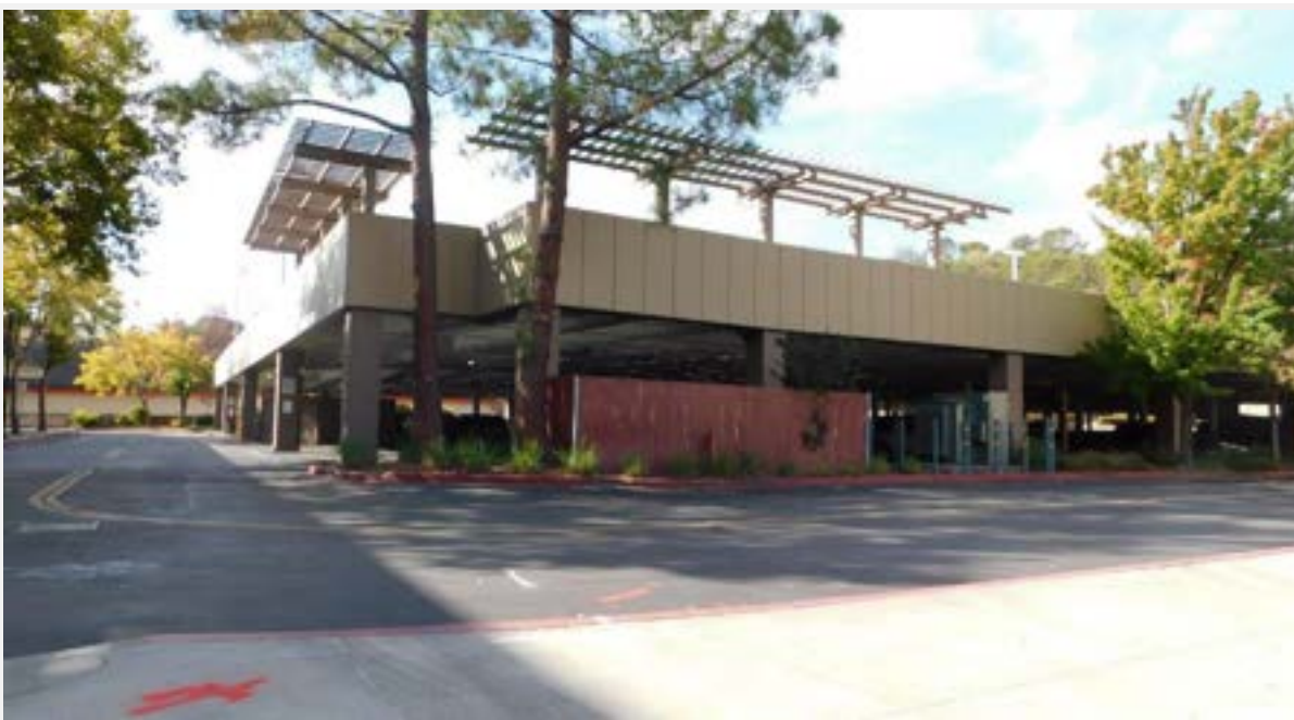
Photograph 18. Parking Garage: West and north elevations, view to southwest (DSCN9423)
