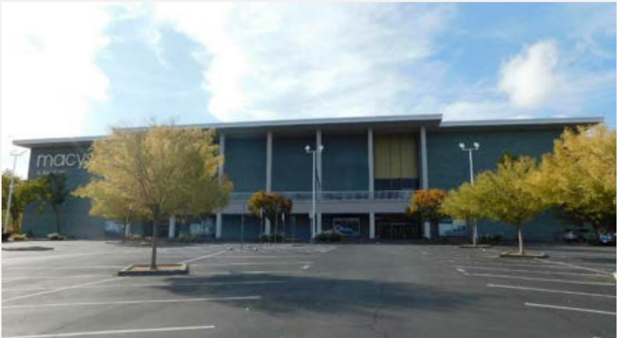
Photograph 3. Emporium: main (north) elevation, view to south (DSCN9373)
