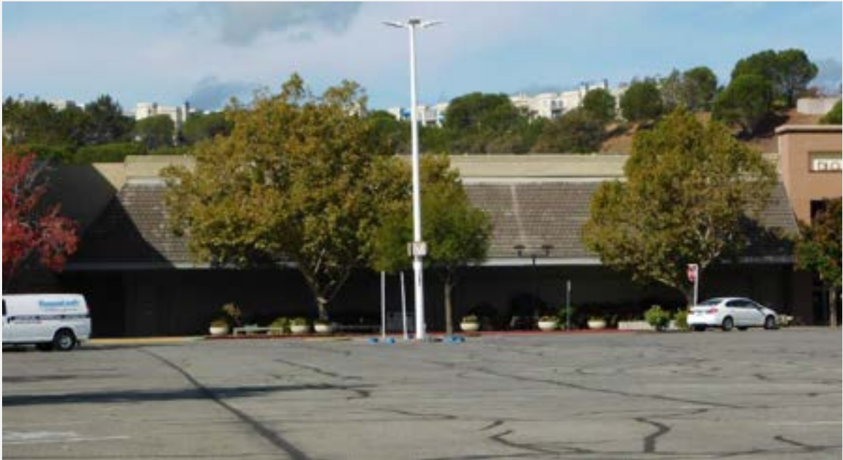
Photograph 9. Northgate Mall Unit 5: East (main) elevation, view to northwest (DSCN9504)
