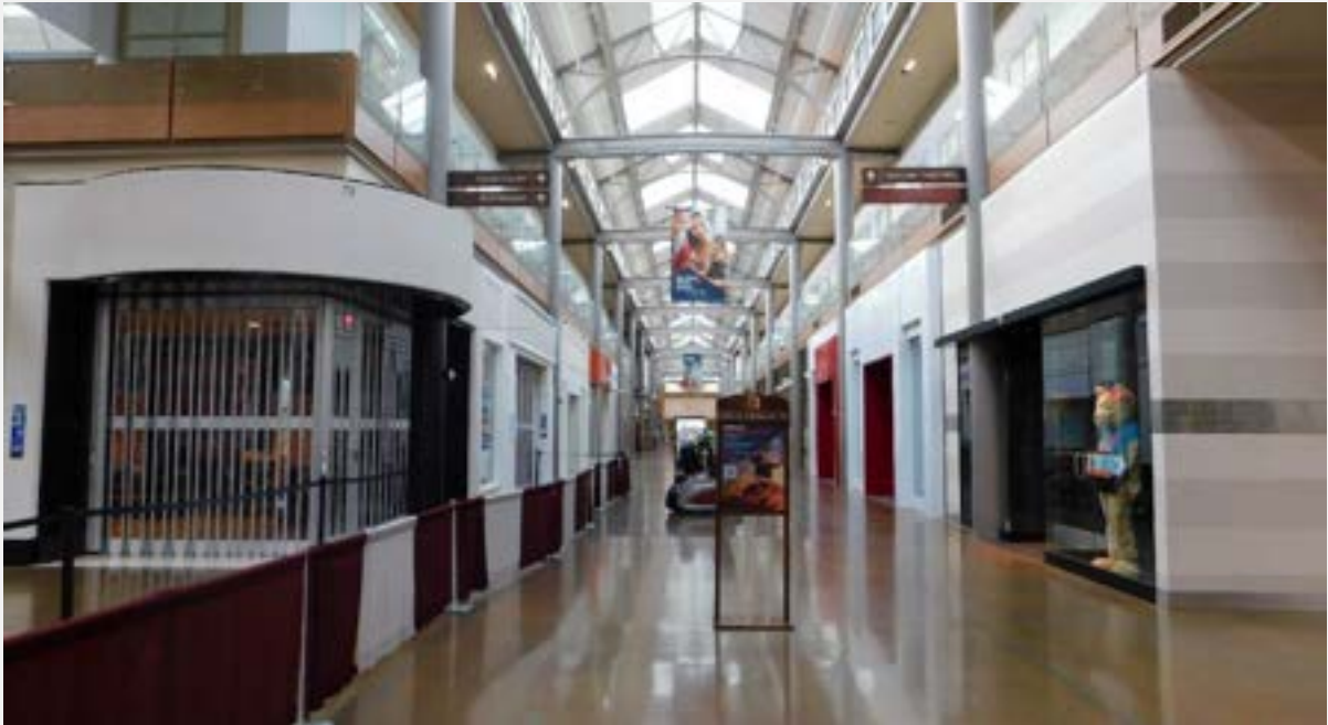
Photograph 16. Mall Enclosure: Detail of enclosure structure, view to south (DSCN9393)
