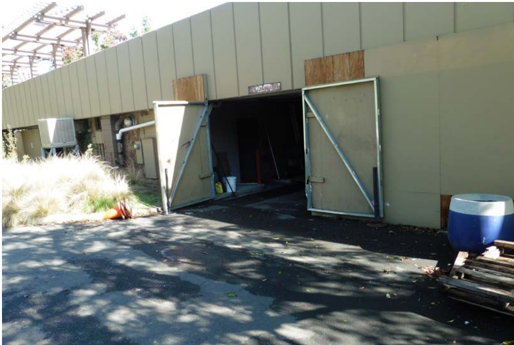
Photo 22: Mall maintenance shop under west side parking garage at Northgate Mall.
