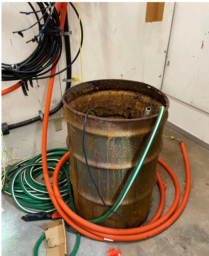
Photograph 19. Empty drum, former Sears basement.
