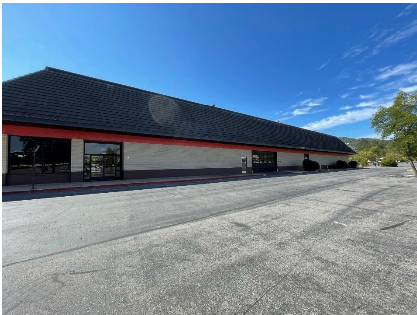
Photograph 1. Former Sears Auto Center building (northside).
