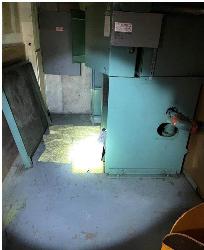
Photograph 20. South freight elevator equipment room, former Sears basement.
