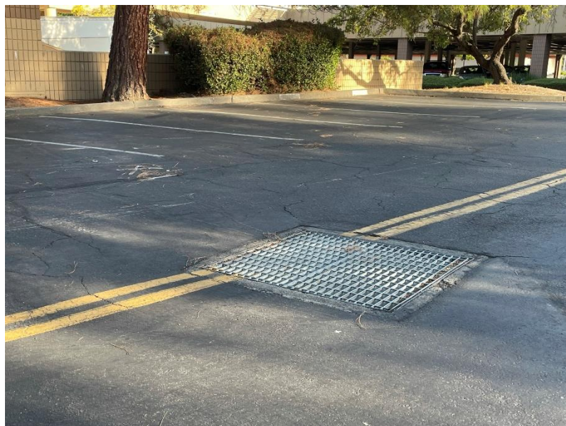
Photograph 45. Example storm drain catch basin in the parking lot.
