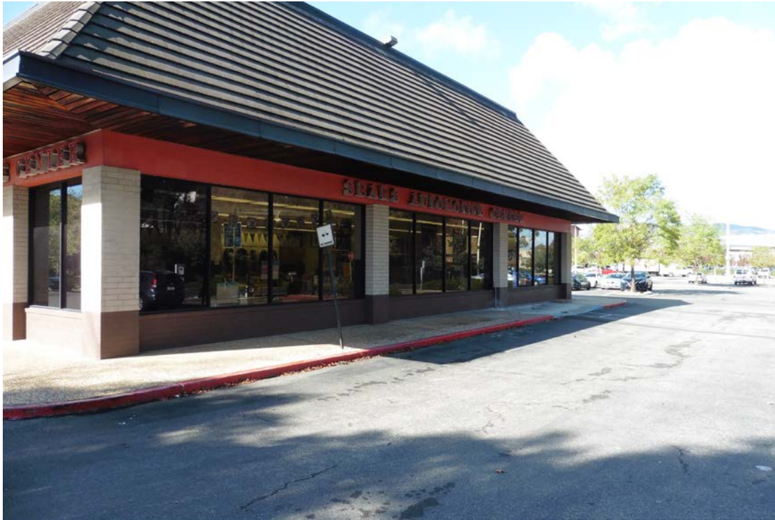
Photo 7: Sear's Automotive Service Center southeast corner of Northgate Mall Property.
