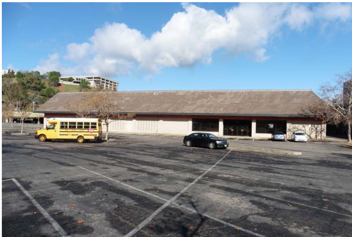
Photo 6: Vacant former Sears appliance service center. Camera facing north.
