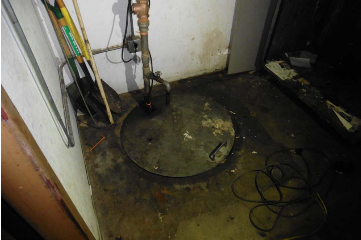
Photo 18: Sump in Sear's basement area.
