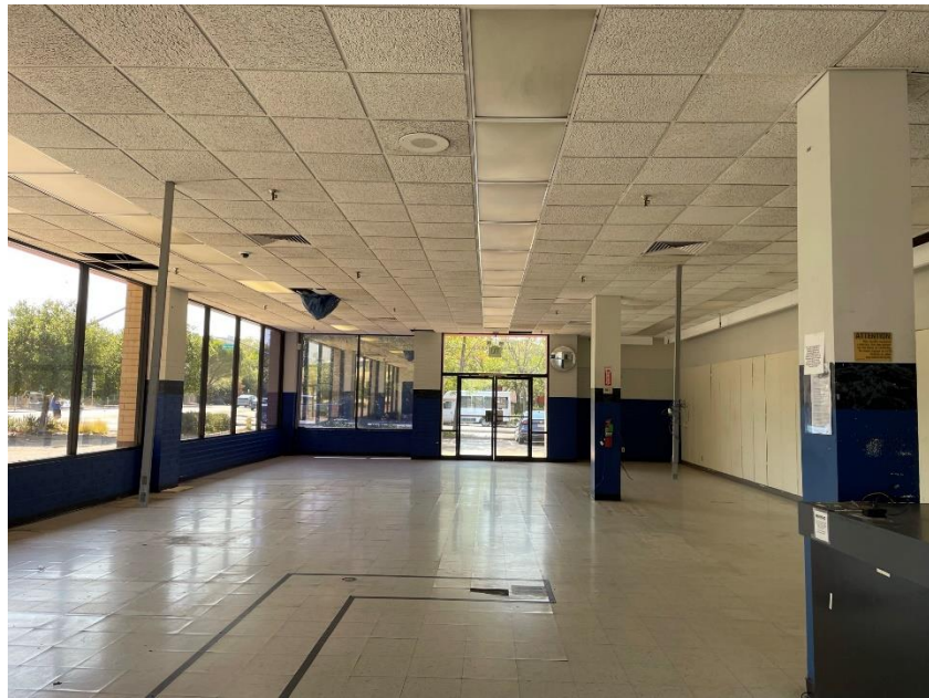
Photograph 3. Front room of former Sear Auto center facility.
