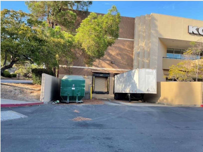
Photograph 34. Kohl's loading dock and trash compactor.
