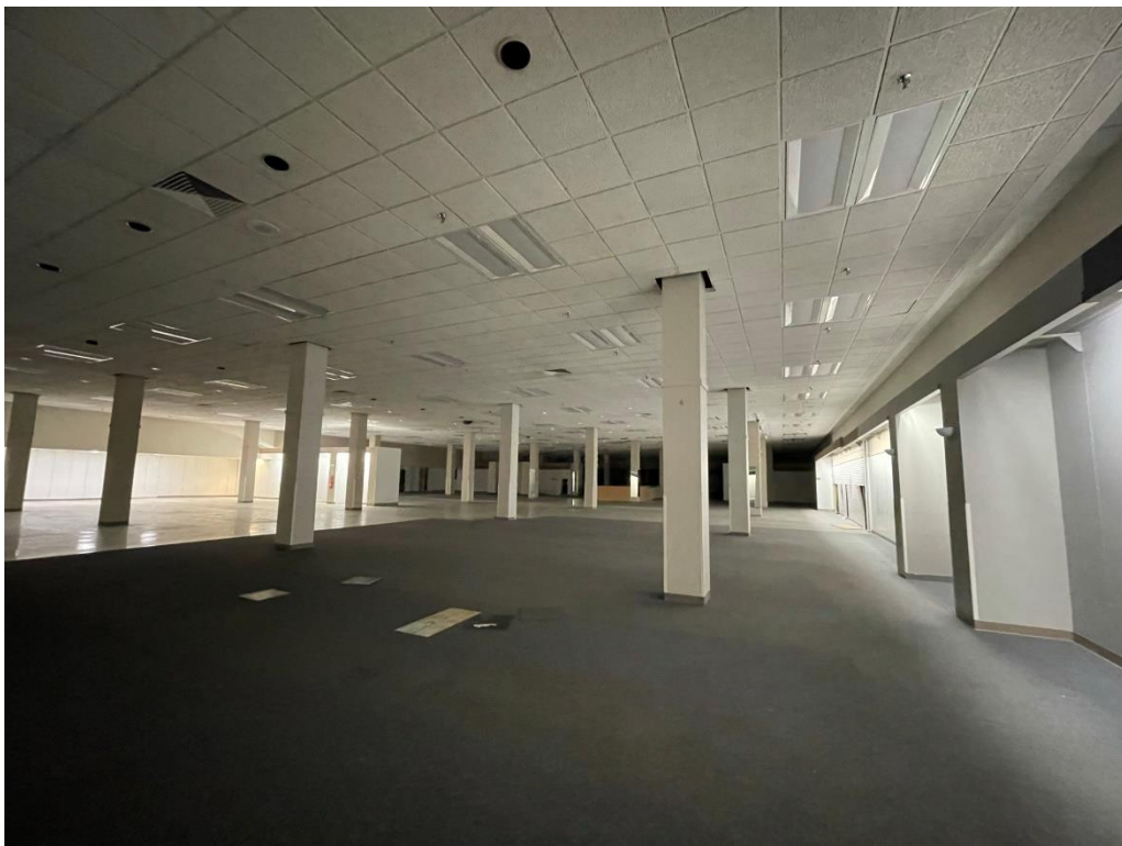
Photograph 23. Former Sears second floor retail space.
