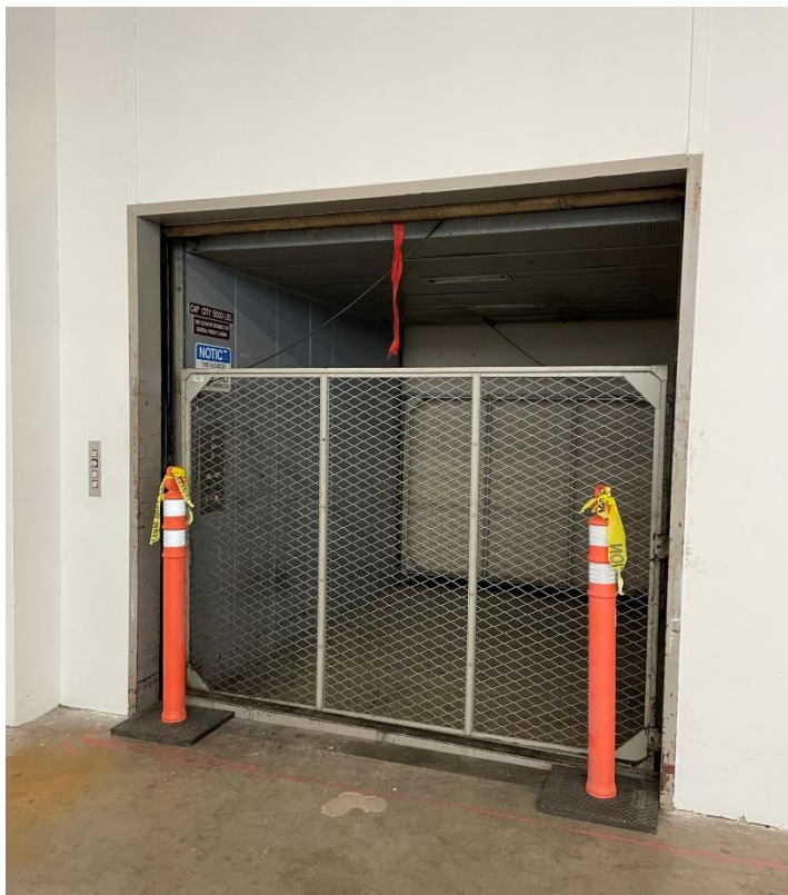
Photograph 17. North freight elevator, former Sears basement.
