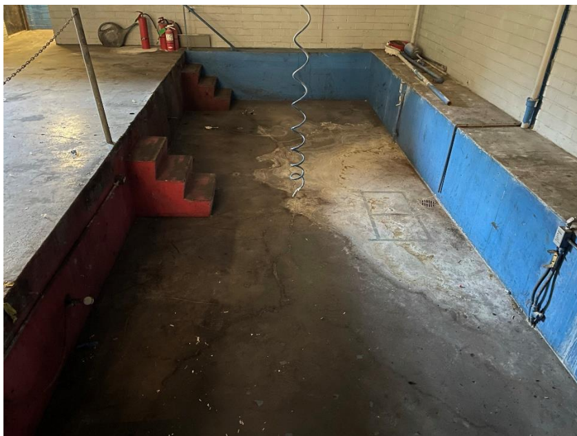
Photograph 6. Sunken work area at northwest corner of auto shop floor.
